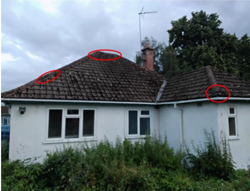
Photo 2. Northern elevation of 11 Sapcote Road, with gaps noted at the ridge, hips eaves and roof slope.
