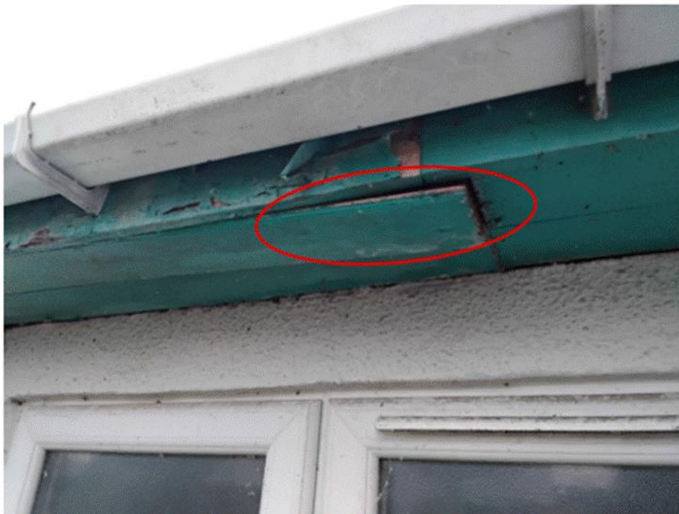
Photo 3: Access point into the soffit
