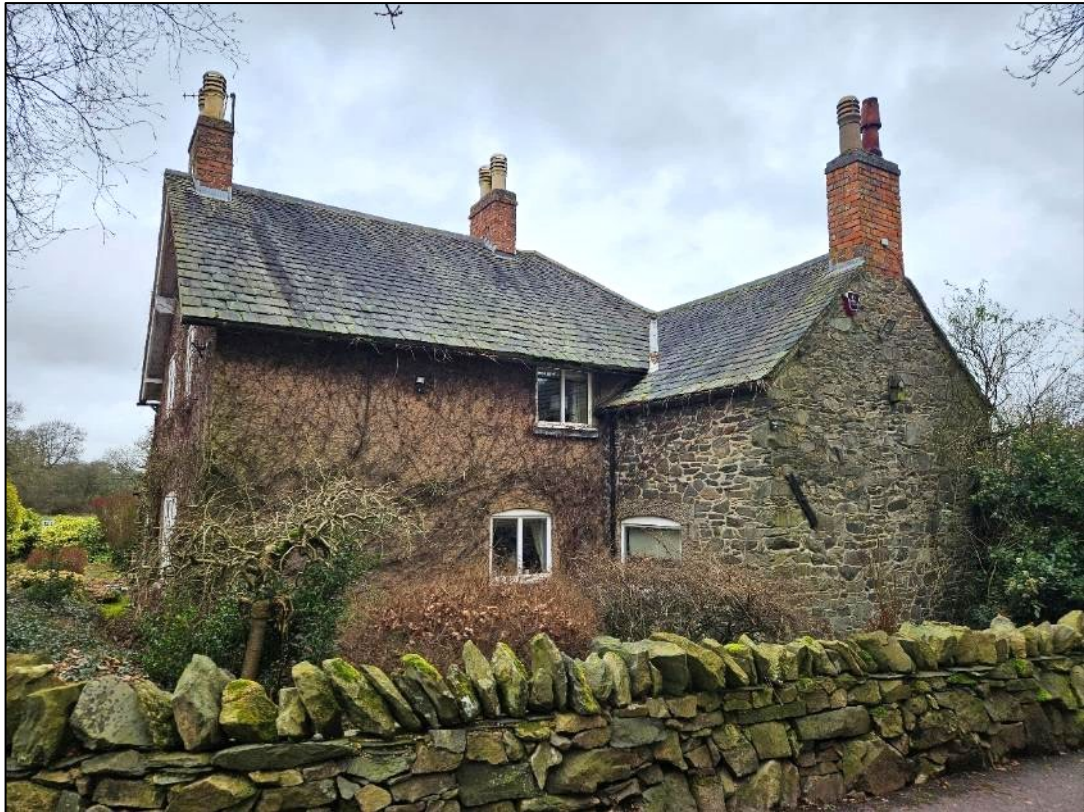
Photo 2. View of Weaver's Cottage, south-east elevation, from Cottage Lane (looking north)
