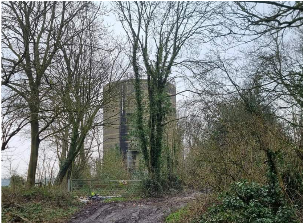
1.9 – Site entrance pre-purchase, securely gated and locked. Signage clearly restricting unauthorised access
