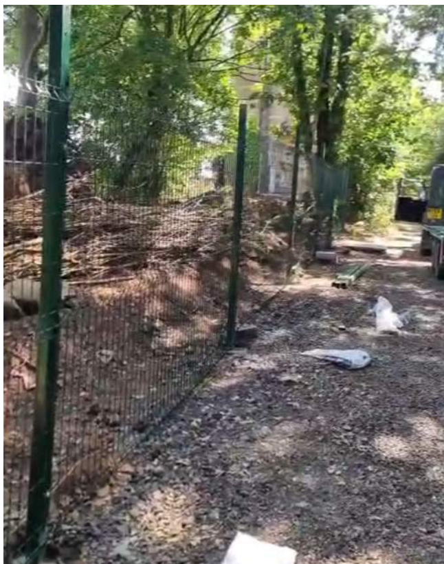
1.6 New Security Fence – metal boundary fencing installed post-purchase
