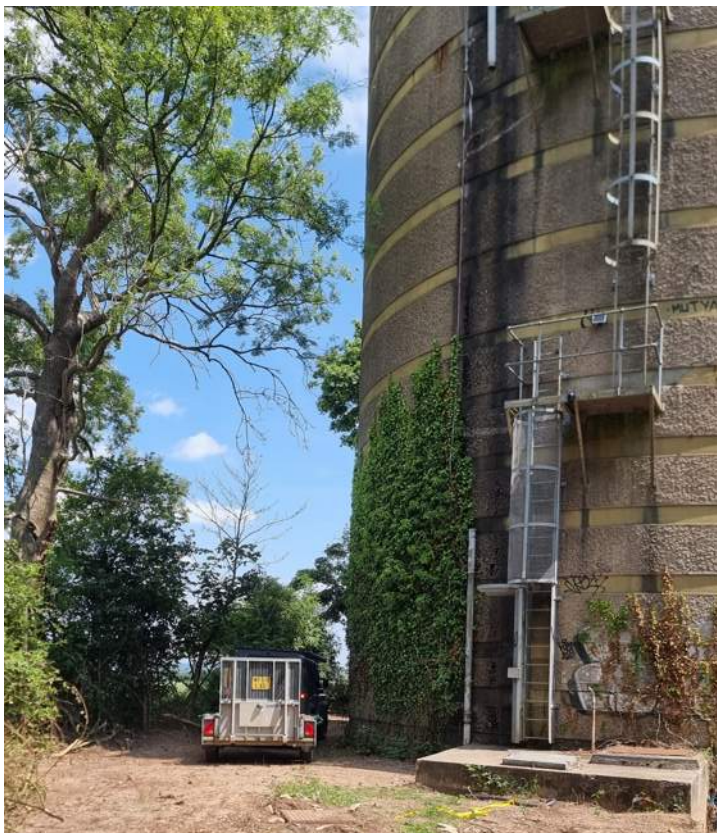
1.5 Water Tower and Yard (July 2025) – active storage in progress
