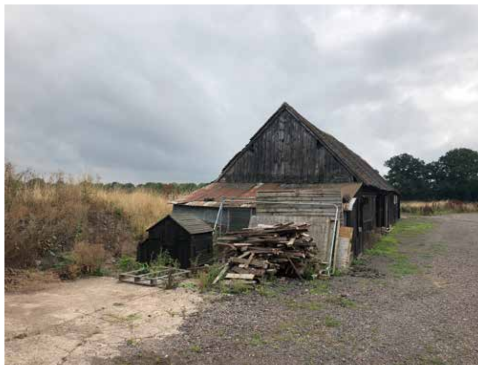
Rear of workshop buildings with earth mound
