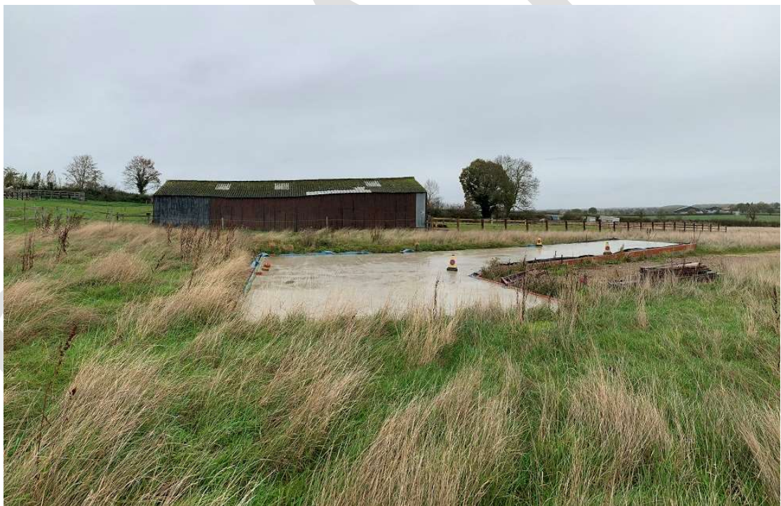
Figure 23: The stable foundations at the north-west side of the PDA
