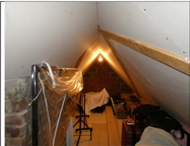
Photograph 21. The western section of enclosed roof void (view to west)
