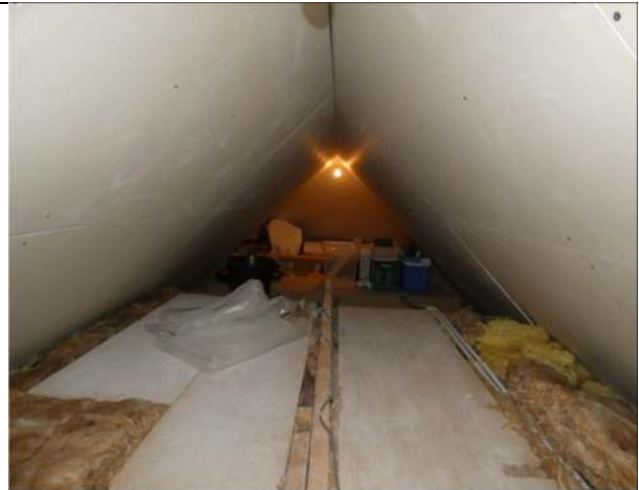
Photograph 26. The section of enclosed roof void within the easternmost gabled projection to the south
