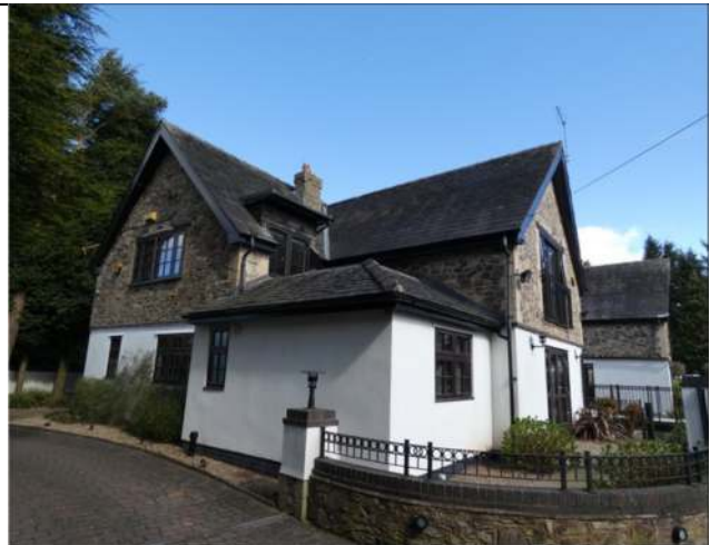
Photograph 4. The west elevation of the house
