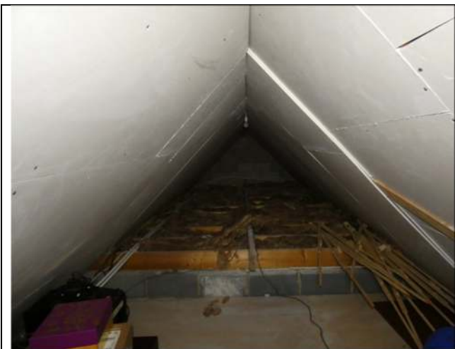
Photograph 23. The section of enclosed roof void within the westernmost gabled projection to the south
