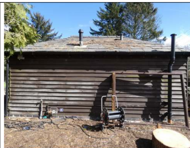
Photograph 33. The west elevation of the outbuilding
