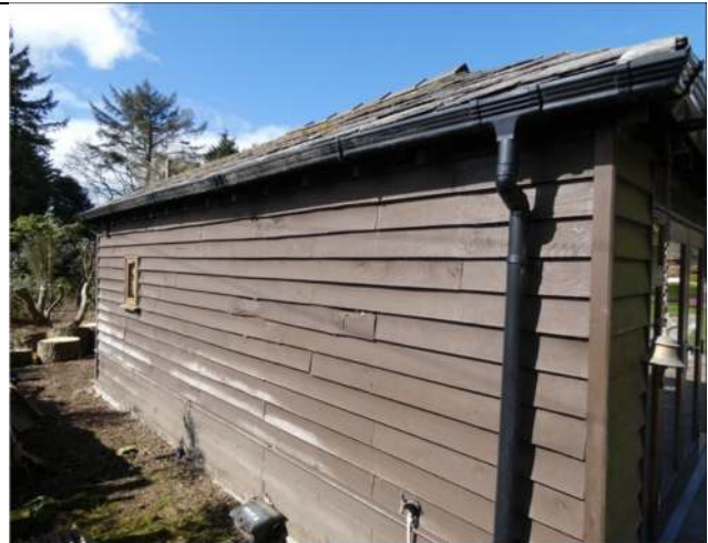
Photograph 32. The south elevation of the outbuilding
