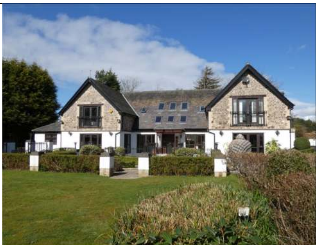
Photograph 5. The south elevation of the house
