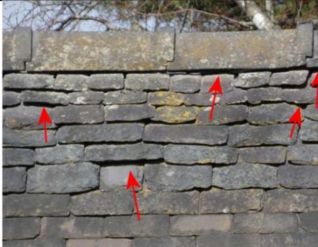
Photograph 7. Example of openings under slates on the main roof of the house
