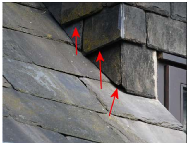
Photograph 12. Example of openings under hanging slates on the north-facing dormer window
