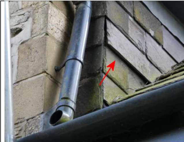
Photograph 13. Example of openings under hanging slates on the south-facing dormer window
