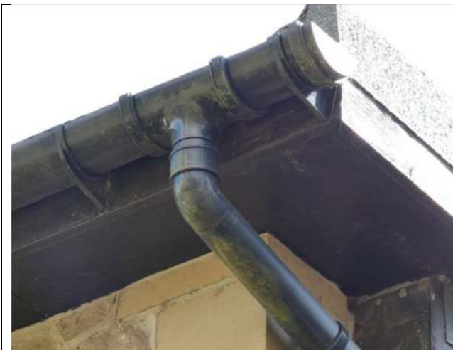
Photograph 15. Example of the soffit and fascia
