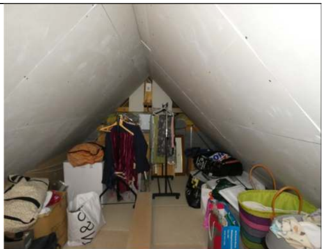
Photograph 24. The eastern section of enclosed roof void within the house (view to west)
