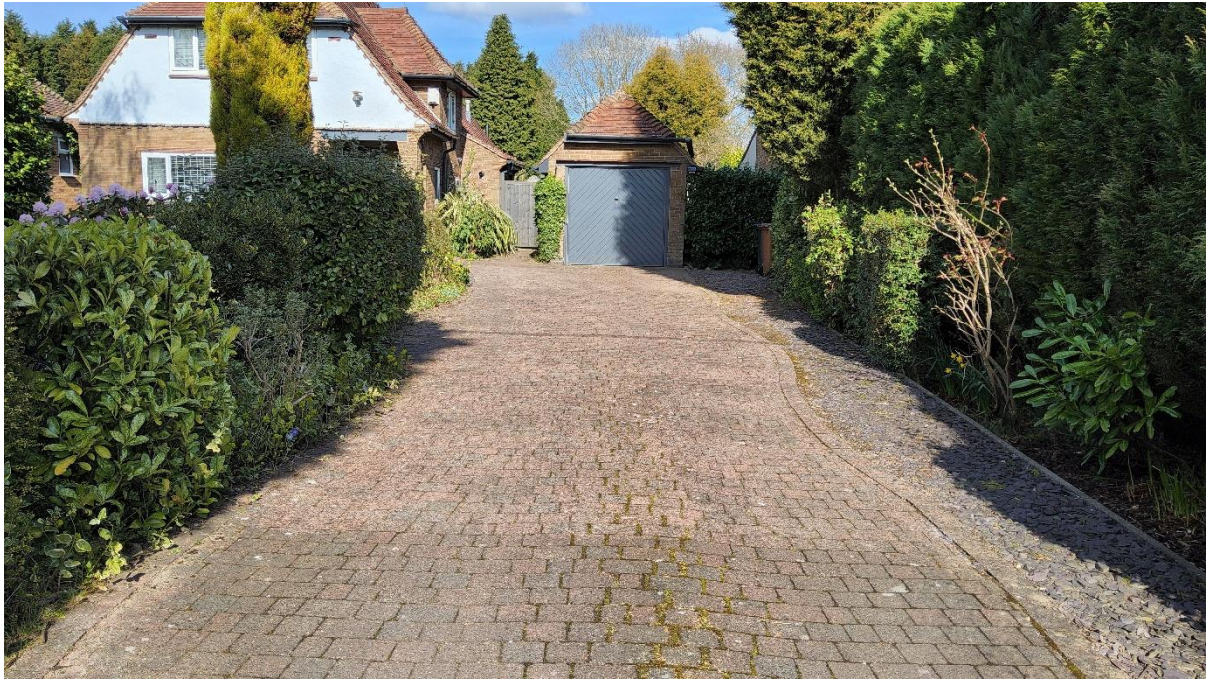
Photo 2. Existing block paving driveway (26871100)
