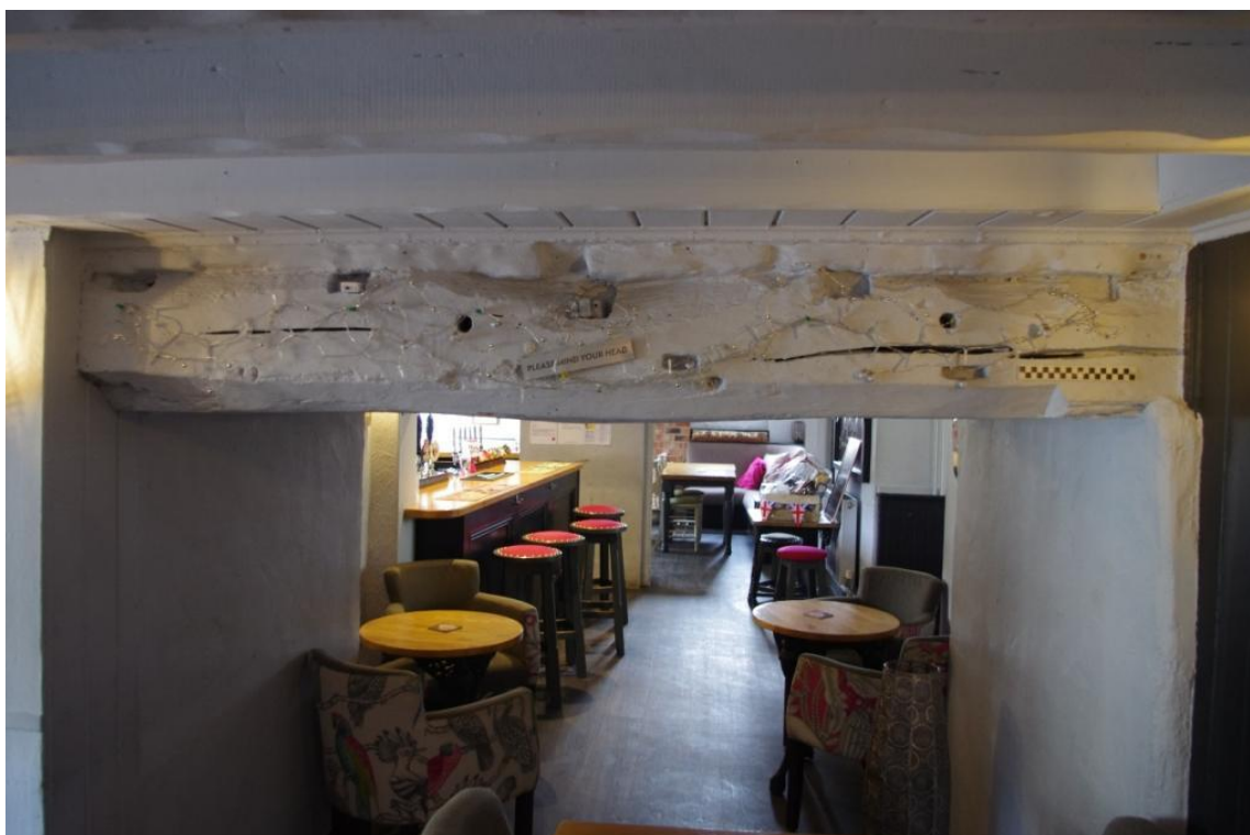
Figure 18 A (4), Fireplace Bressummer (Looking West – North West).
