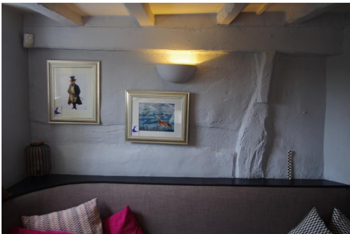
Figure 20 B(1), Framing Visible in Rear Wall (Looking North – North East).
