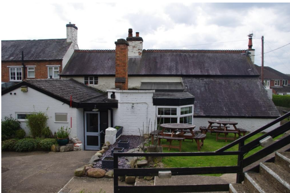
Figure 15 Building A , Rear Elevation at West End (Looking South – South East).
