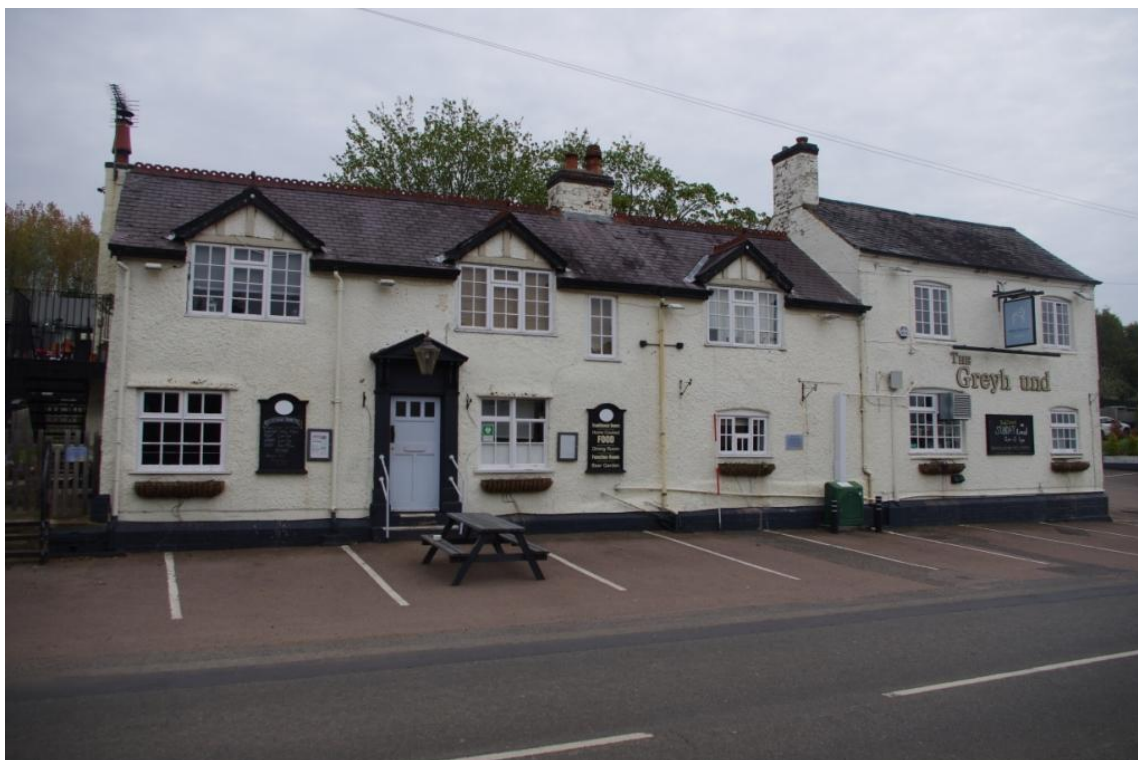
Figure 10 Building A , Principal Elevation (Looking North – North East).
