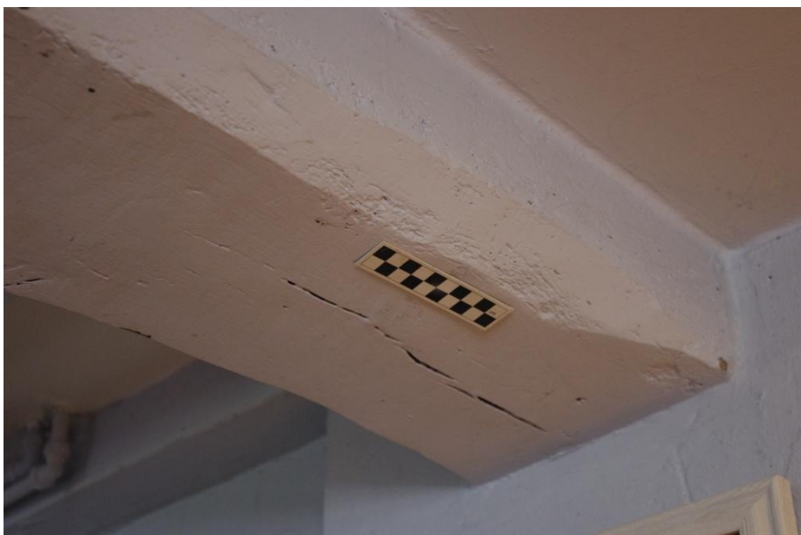
Figure 19 A (1), Chamfered & Stopped Bridging Beam (Looking North East).
