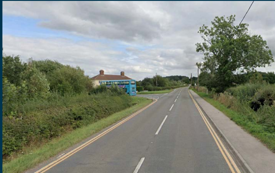
Figure 2.7- Access from A444 from west
