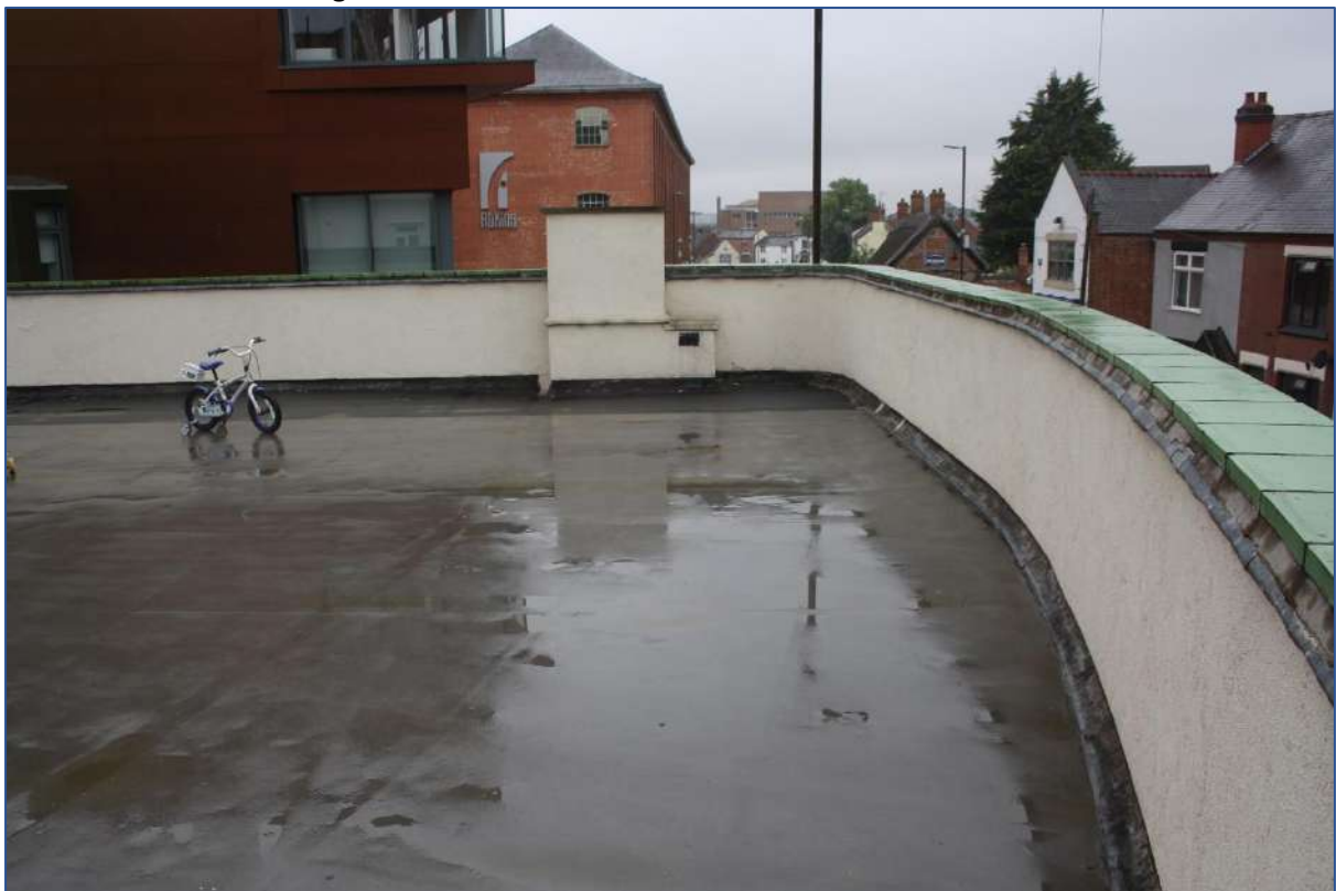
Plate 67: Roof area 27 looking S/W.
