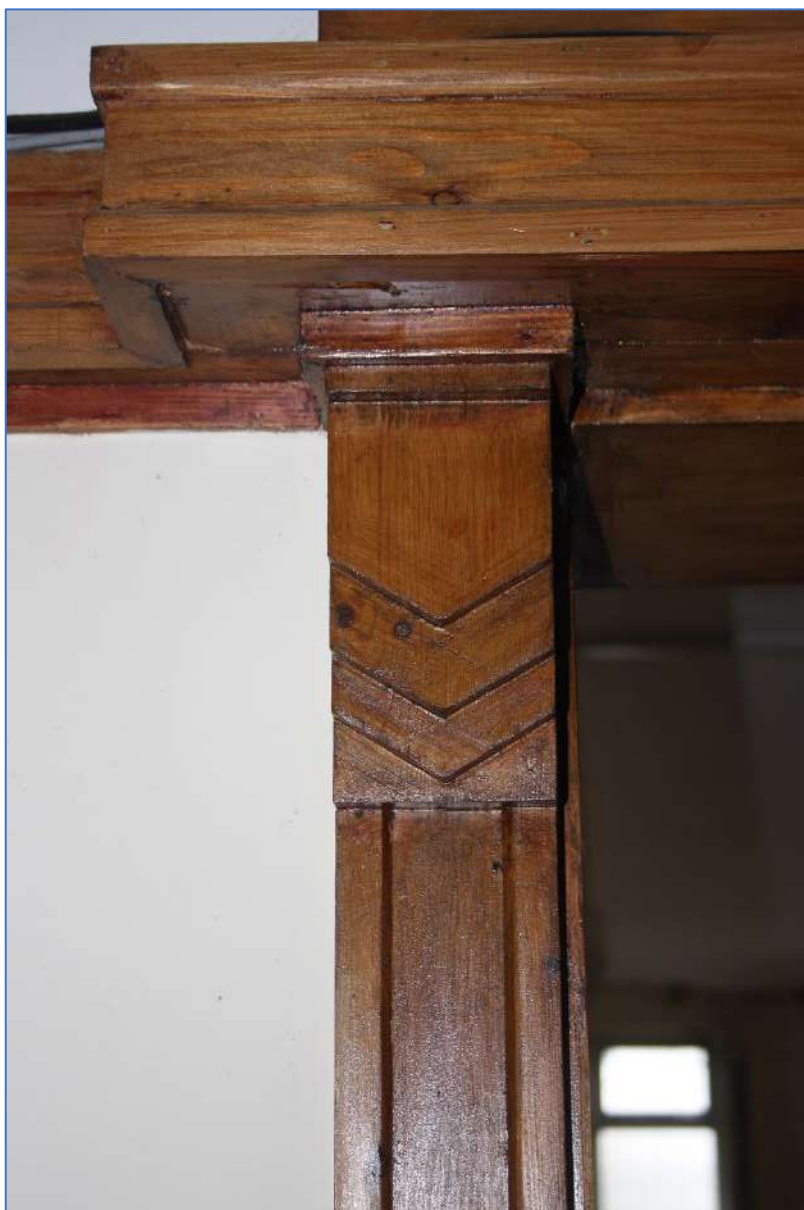
Plate 8: Door frame detail looking N/E.
