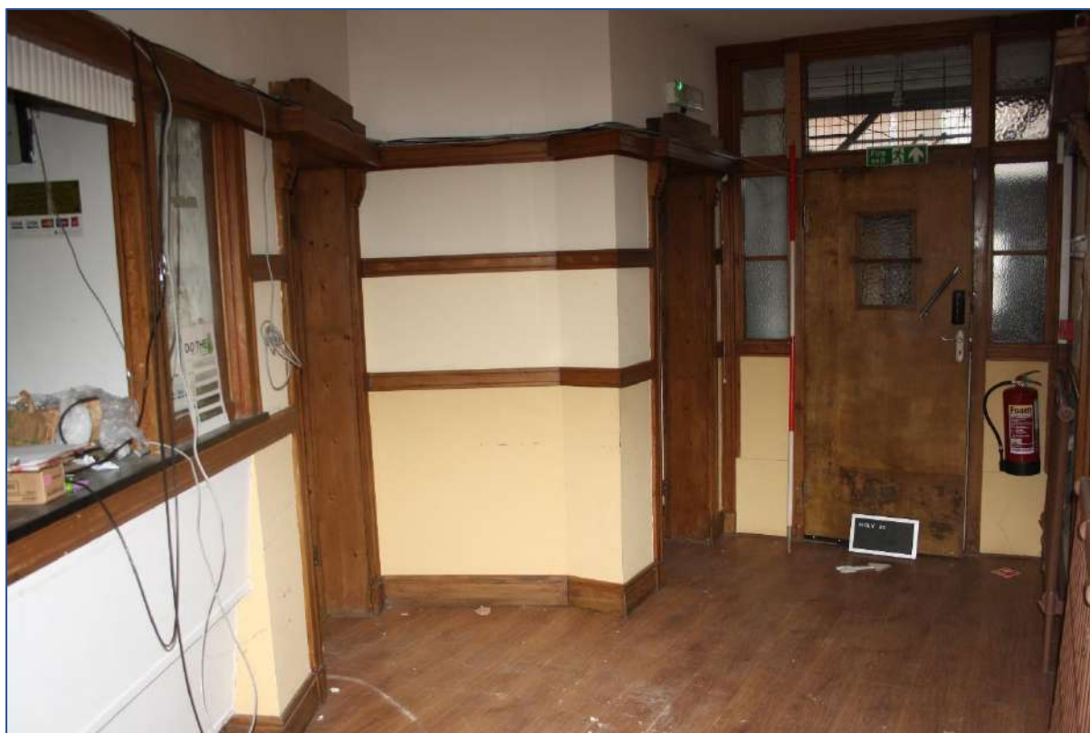
Plate 23: Room 5 Entrance Hall looking N/W.
