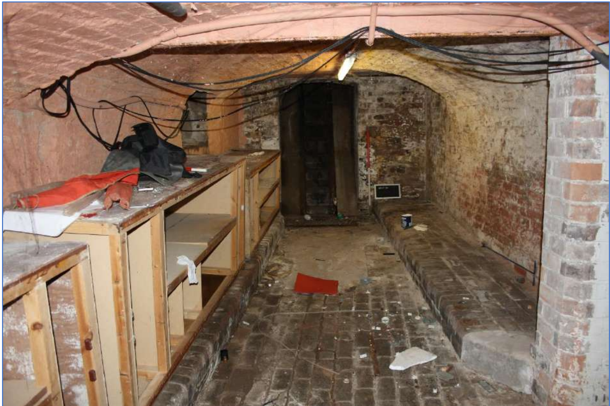
Plate 76: Vaulted brick Cellar A looking south.
