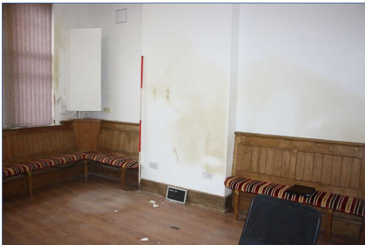
Plate 47: Room 3 looking E.
