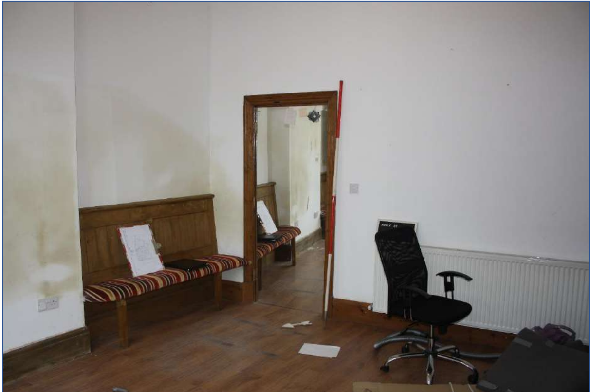
Plate 49: Room 3 looking S/E.
