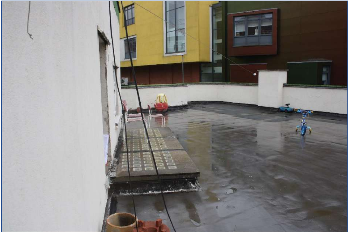
Plate 70: Roof area 27 looking S/E.
