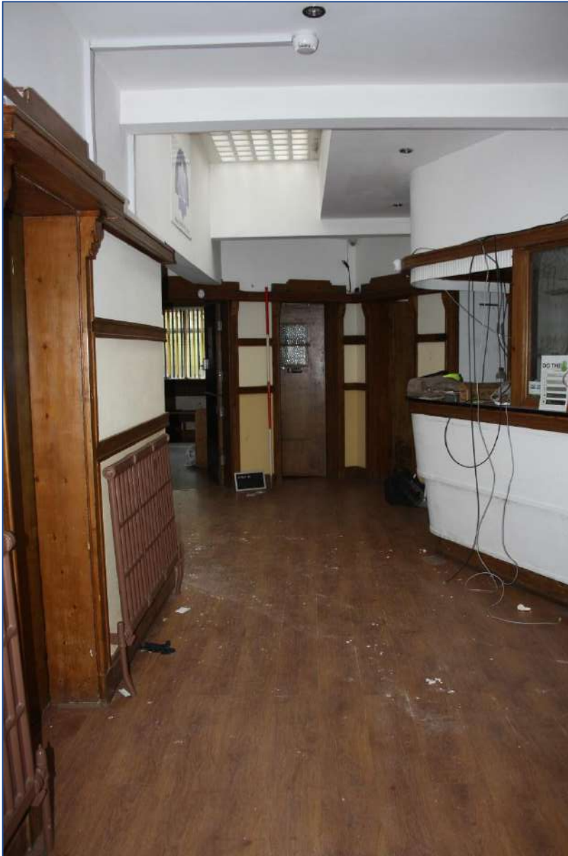
Plate 22: Room 5 Entrance Hall looking S/E.
