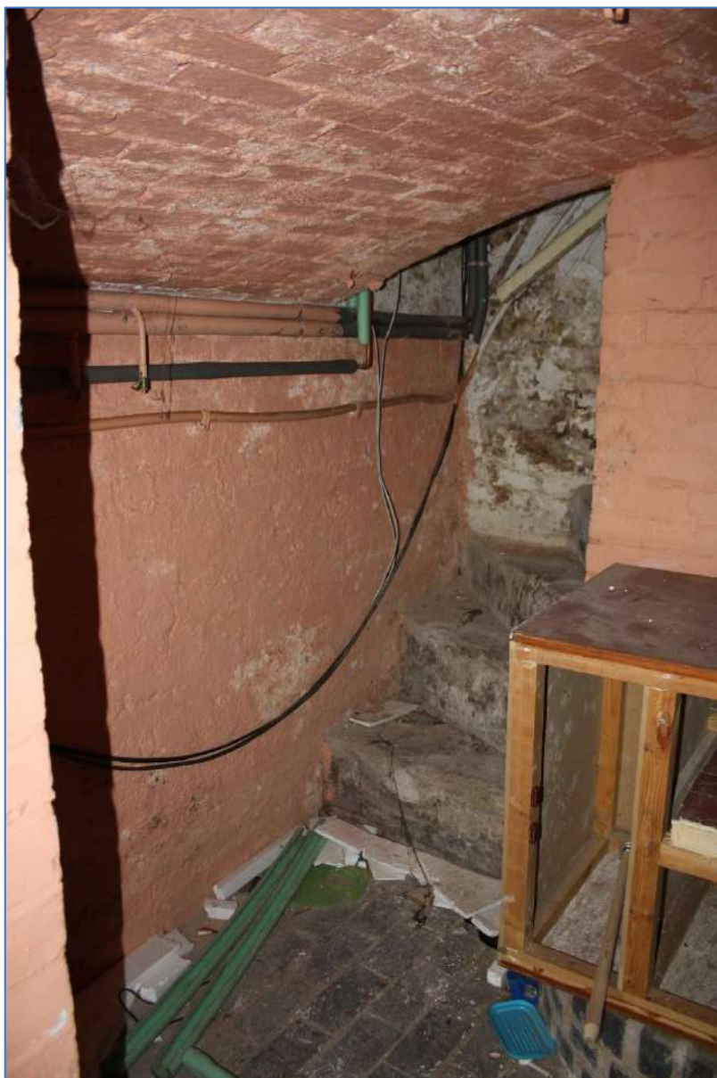
Plate 75: Cellar A steps leading up.
