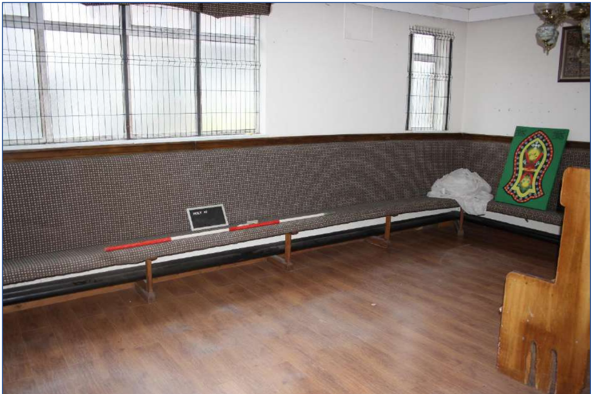
Plate 18: Room 1 looking N.
