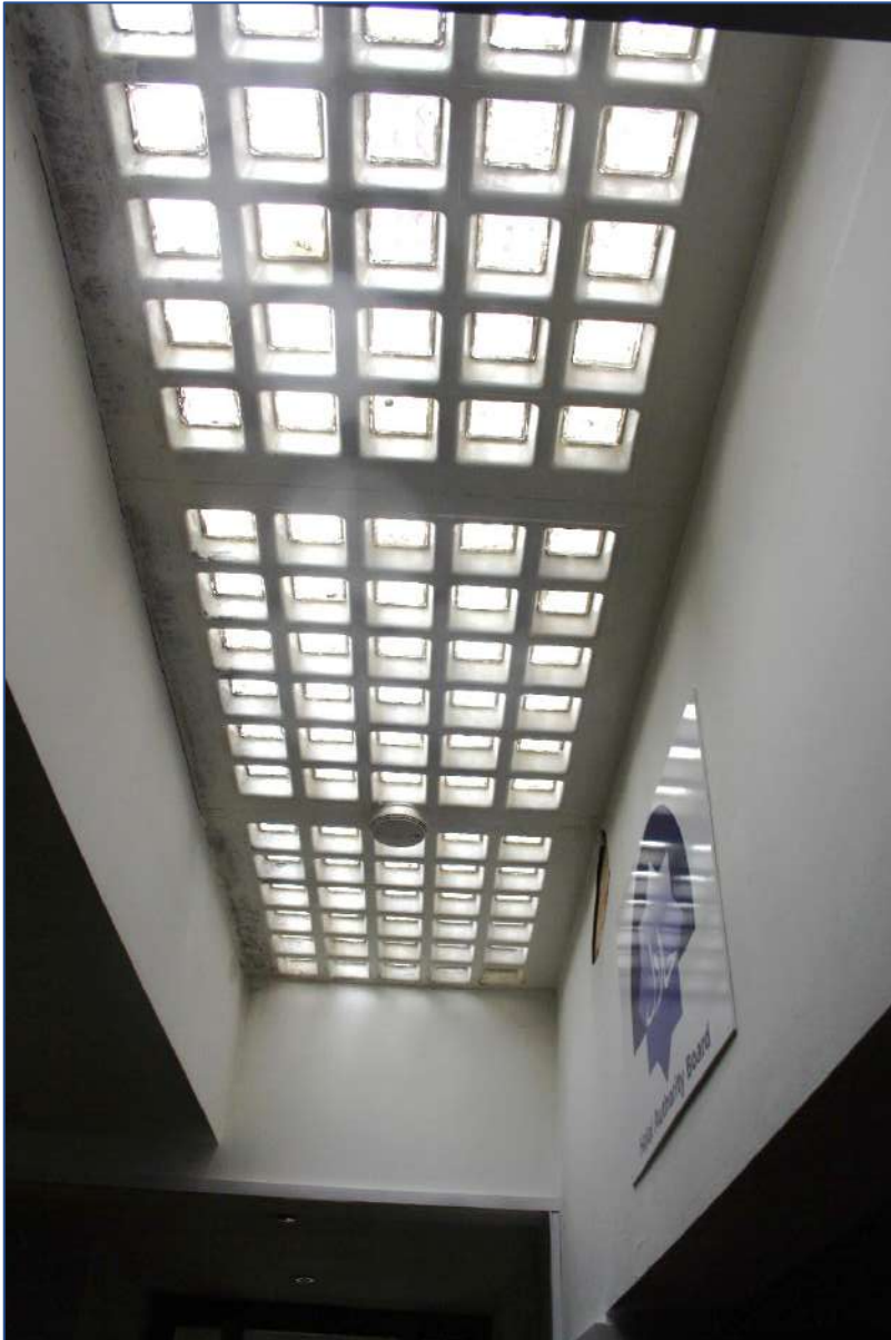
Plate 30: Room 5 ceiling looking N/W.
