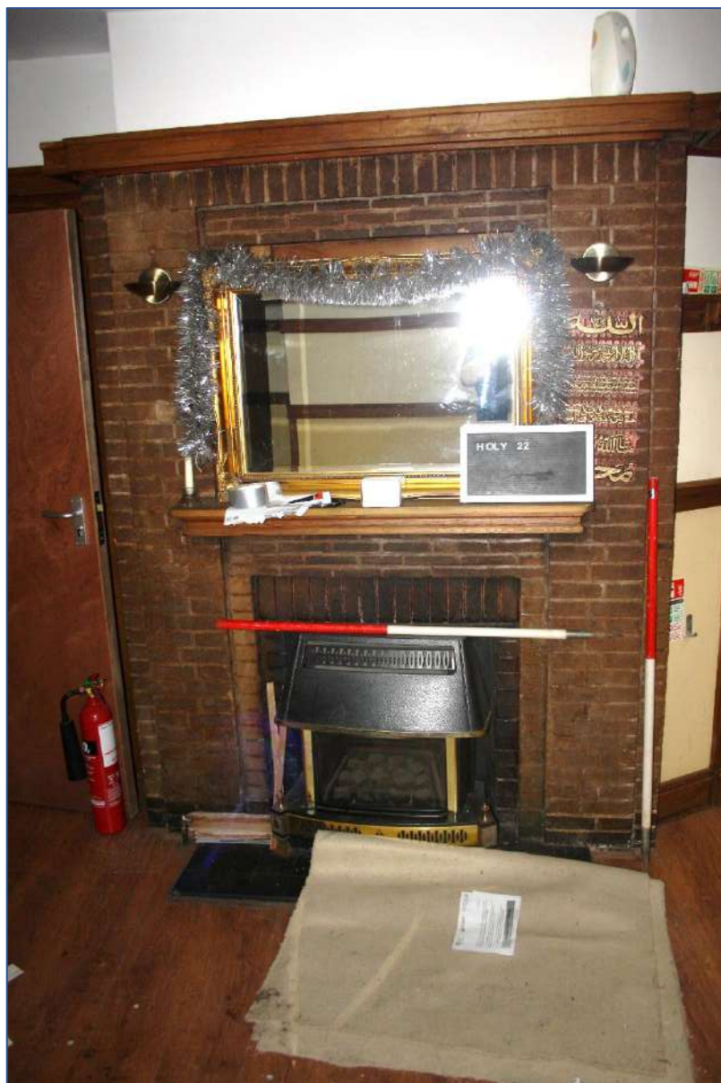
Plate 29: Room 6 looking S/E.
