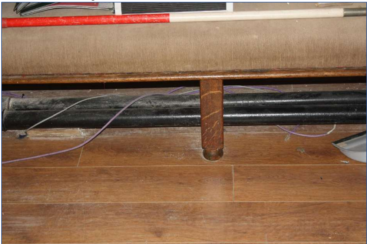
Plate 37: Room 12 seating detail looking S/W.
