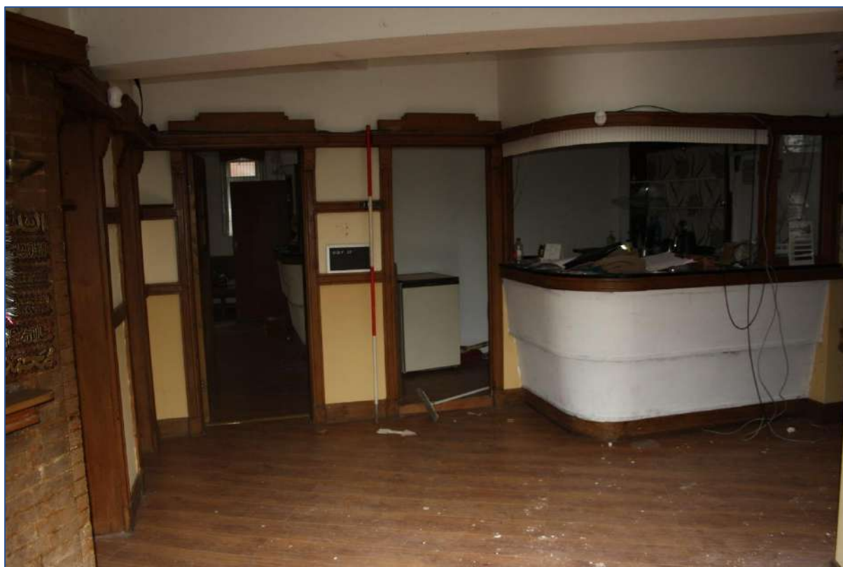
Plate 28: Room 6 looking S/W towards Room 5.
