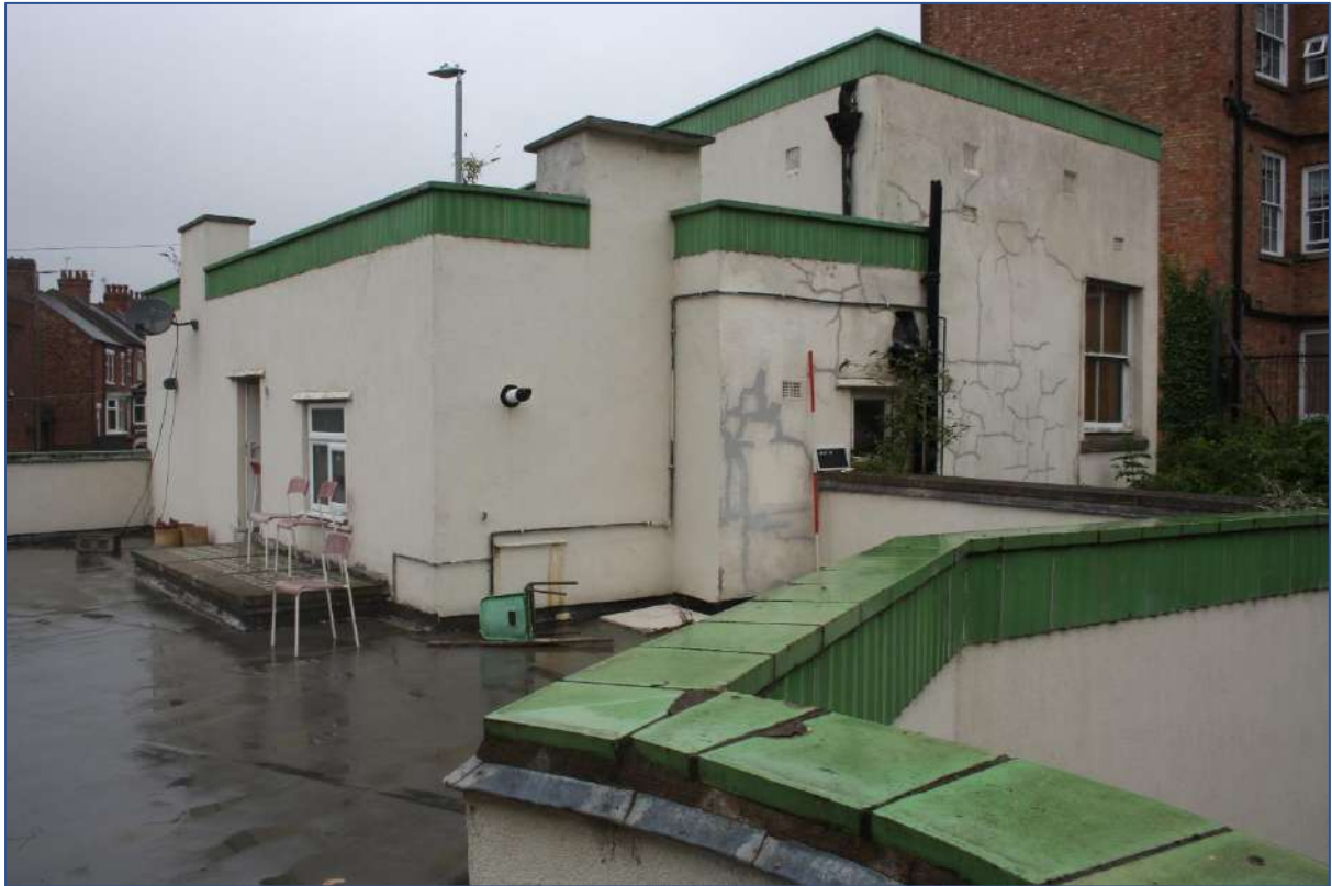
Plate 72: Roof area 27 looking N.
