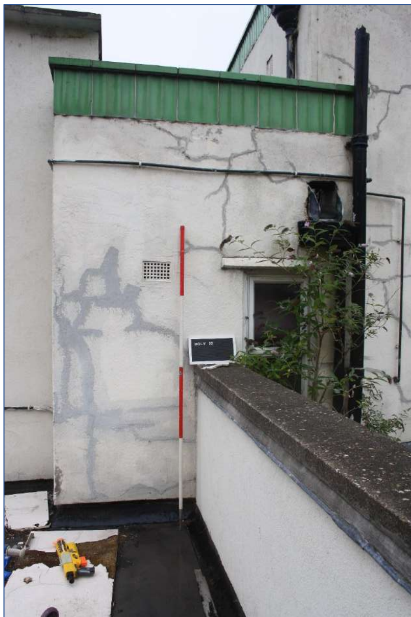
Plate 73: Roof area 27 looking N/W.
