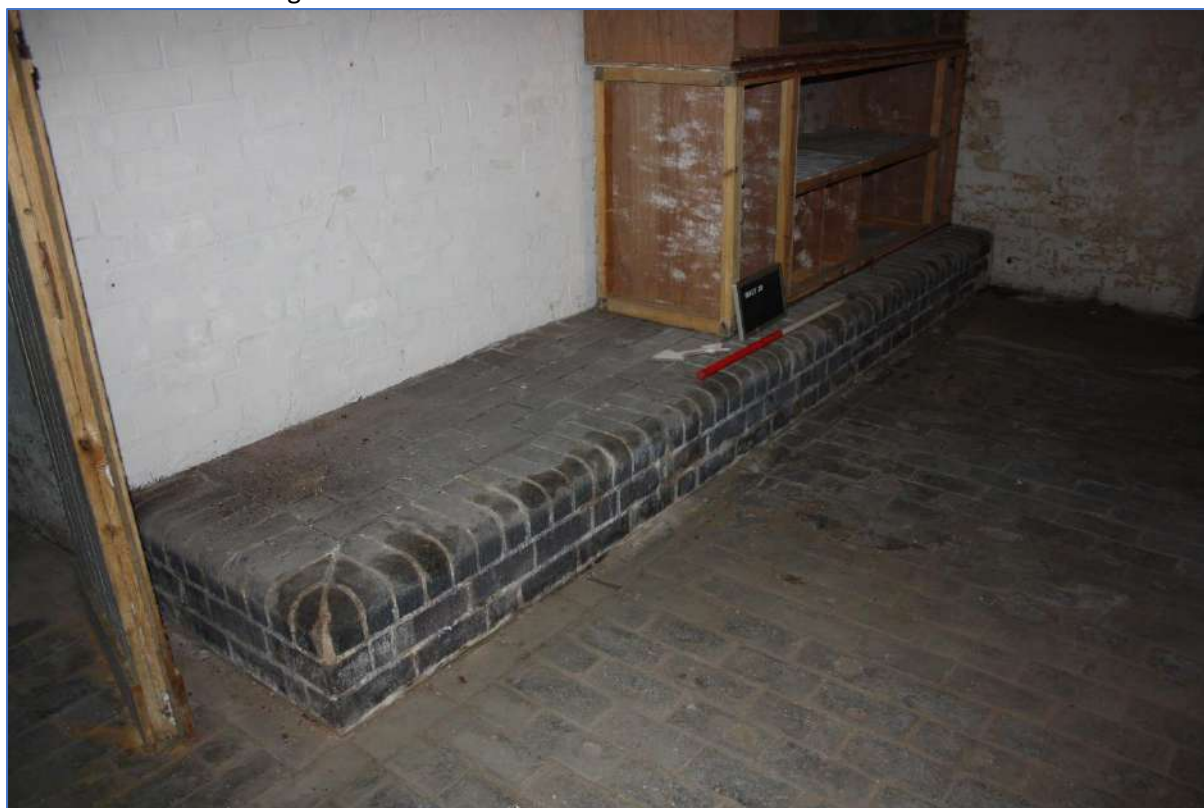
Plate 86: Brick Thrawl in Cellar B looking southeast.
