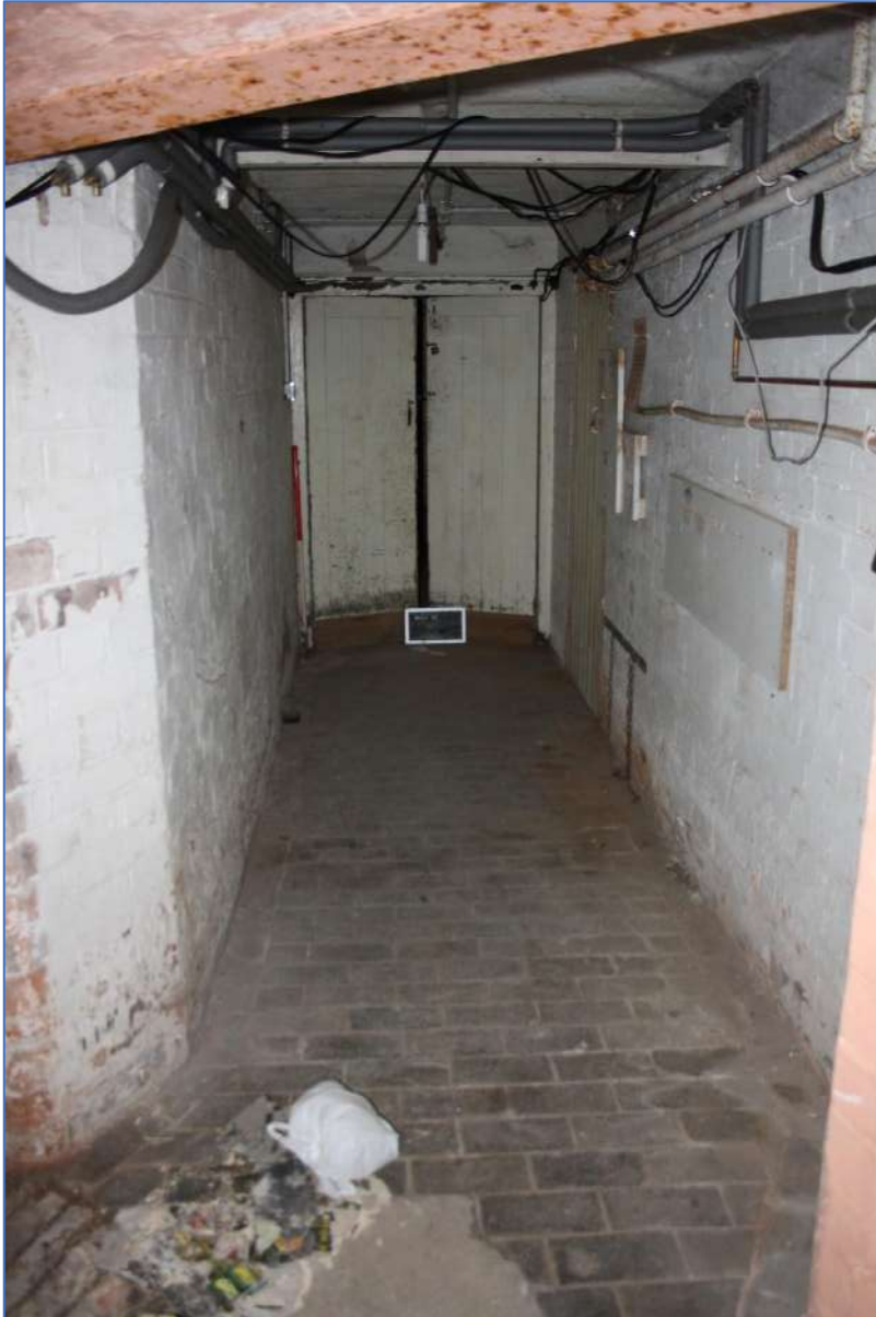
Plate 78: Cellar Corridor looking southwest.
