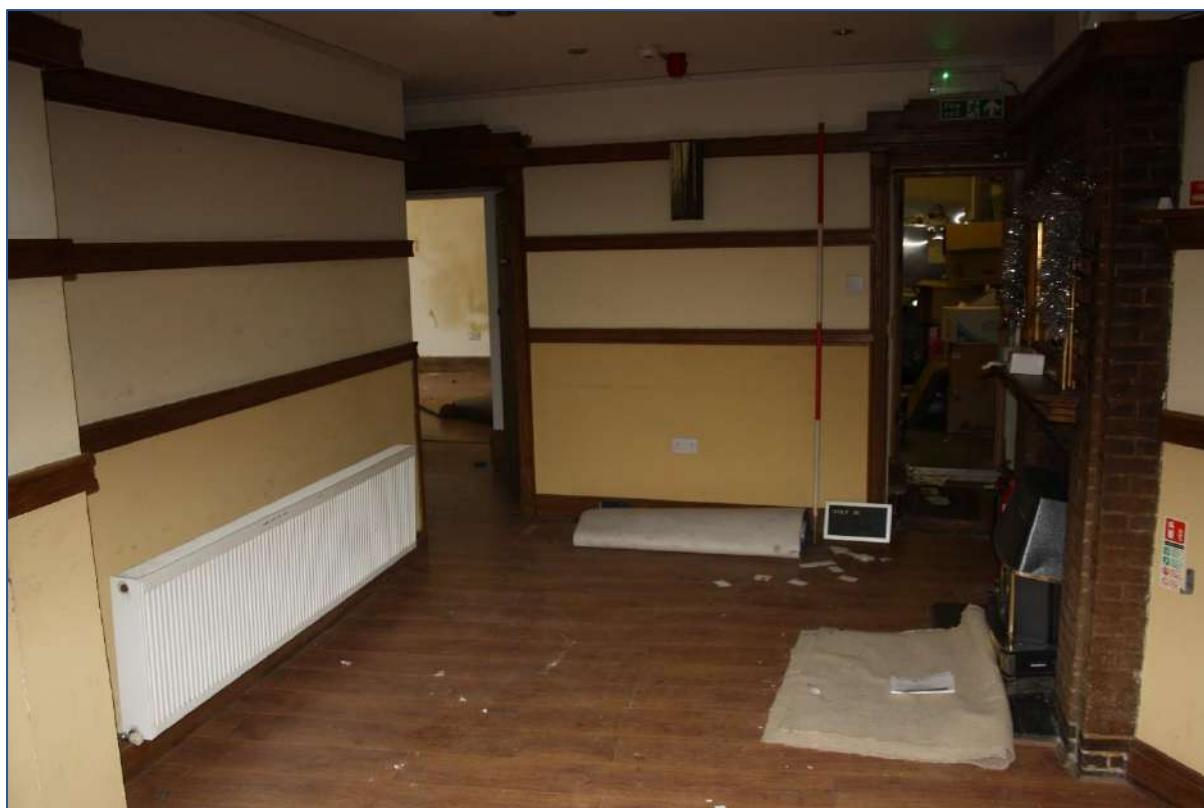
Plate 25: Room 5 Entrance Hall looking S/E.
