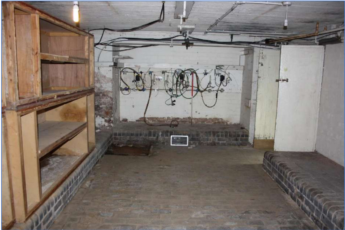
Plate 87: Cellar B looking northwest.
