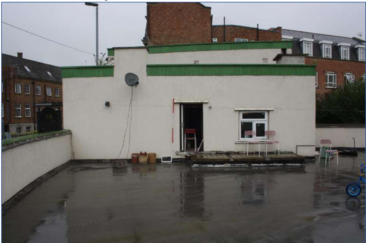
Plate 71: Roof area 27 looking N/E.
