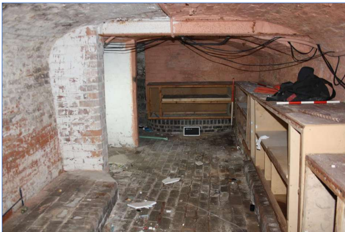
Plate 81: Brick vaulted Cellar A looking north.
