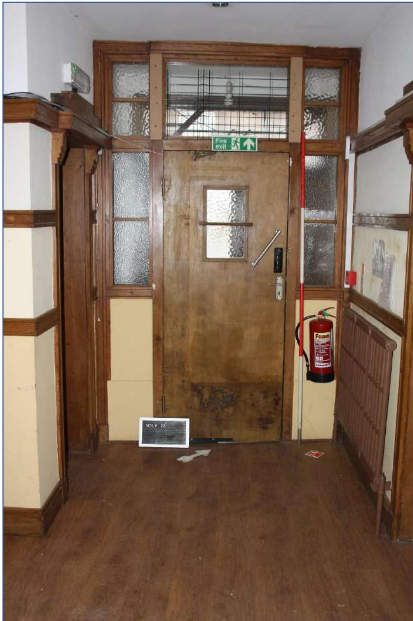
Plate 24: Room 5 Entrance Hall looking N/W to building main entrance.
