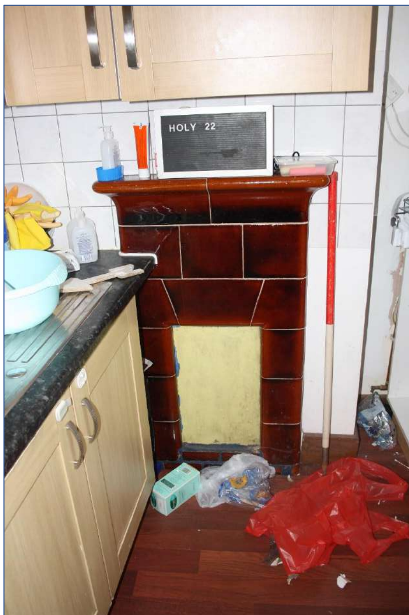
Plate 54: Fireplace in Room 22 looking N/W.
