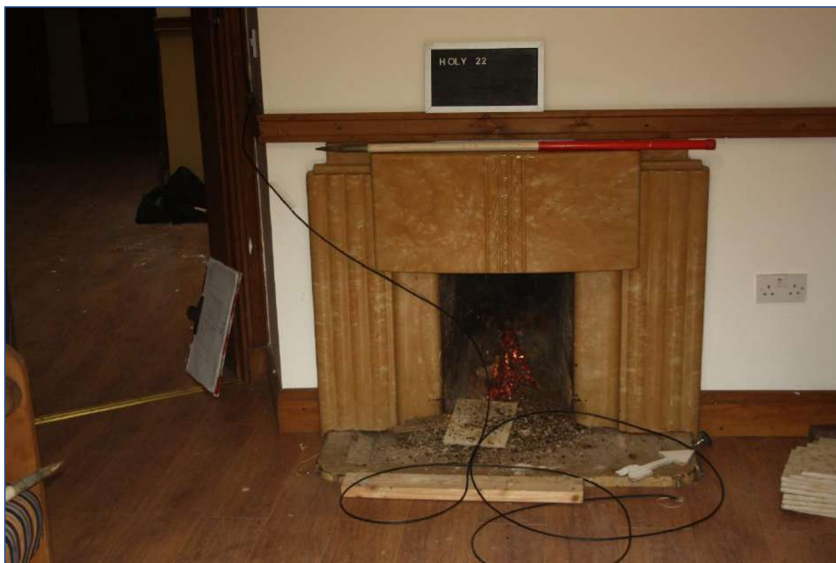
Plate 43: Room 10 fireplace looking N.
