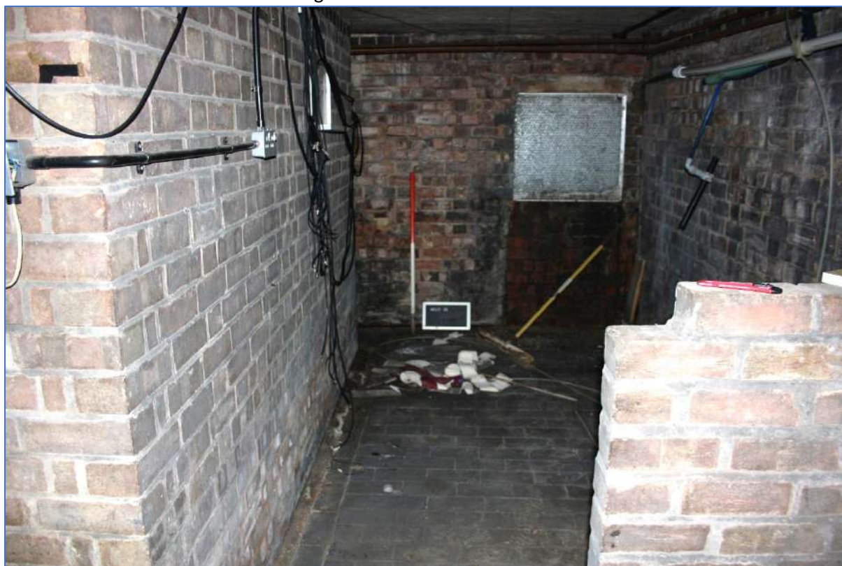
Plate 82: Cellar C looking southwest.
