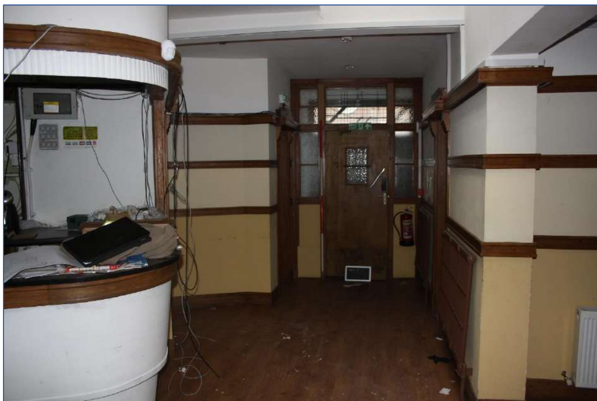
Plate 31: Room 5 looking N/W.
