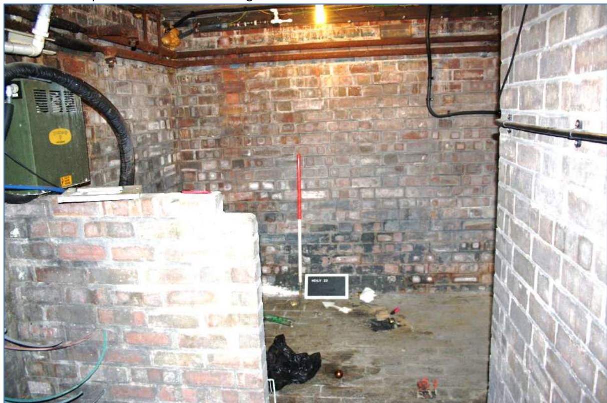
Plate 84: Cellar C looking northeast.
