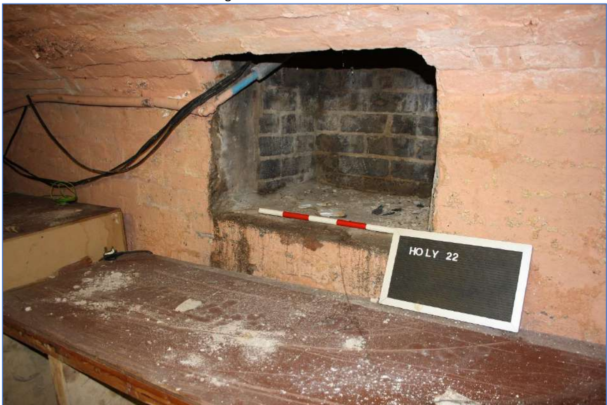
Plate 77: Opening in north south wall looking north.
