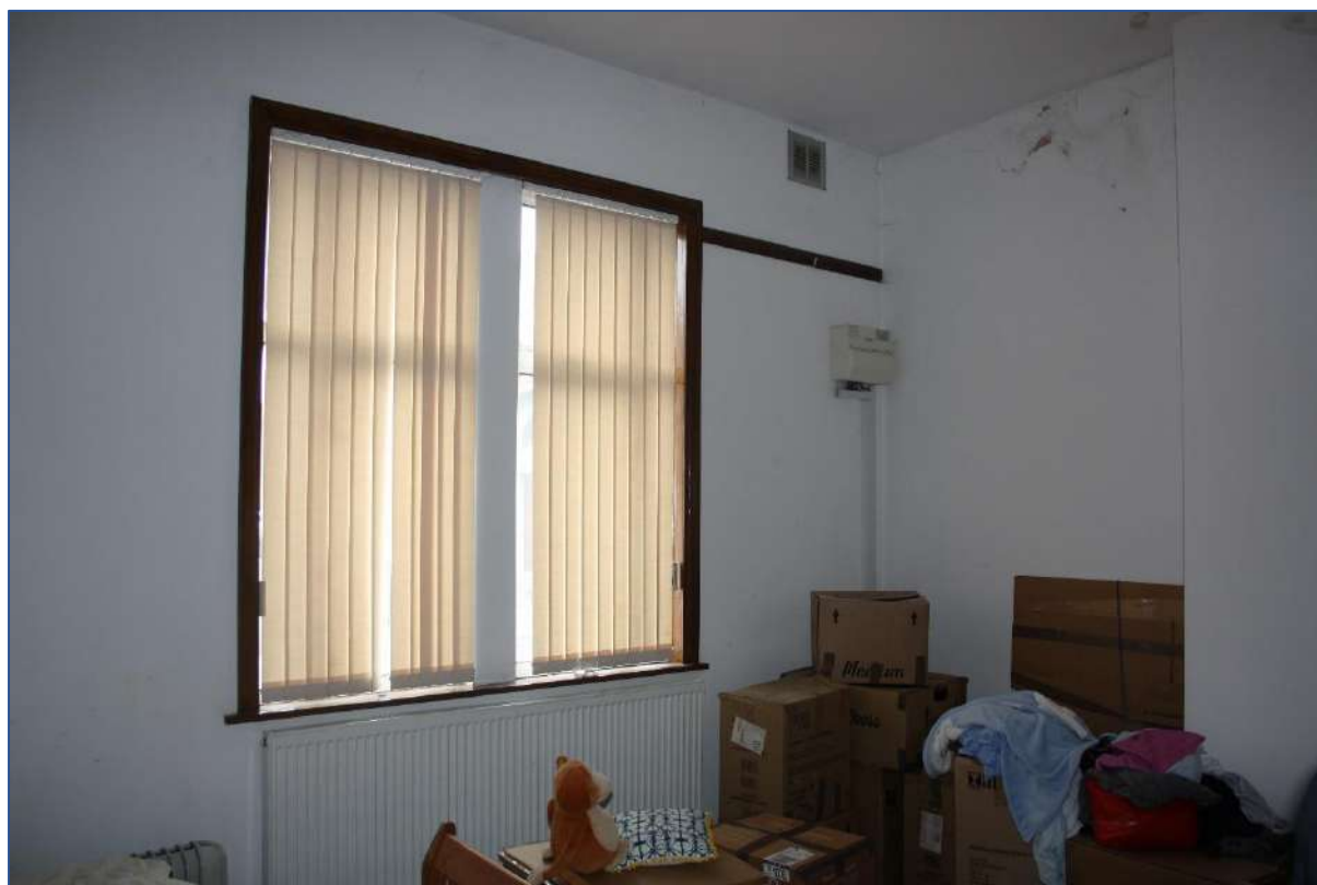
Plate 63: Room 25 looking N.
