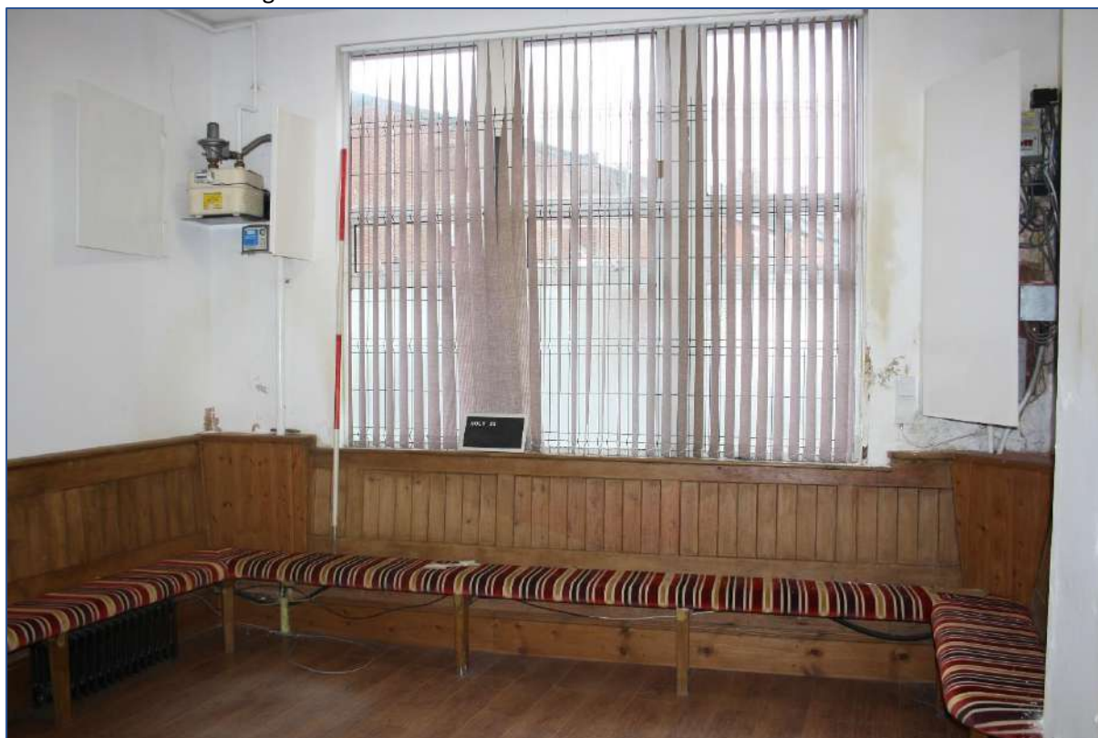
Plate 48: Room 3 looking N/W.
