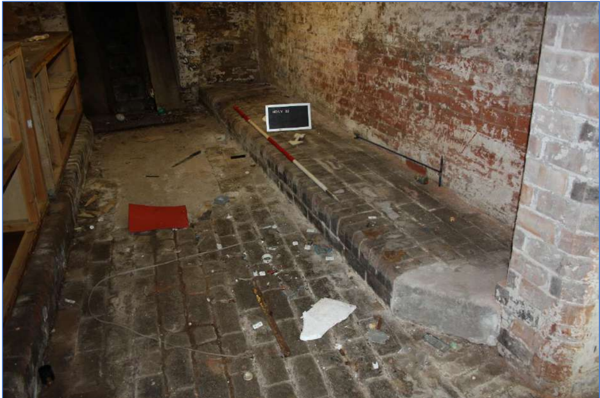
Plate 79: Brick Thrawl in vaulted brick Cellar A looking southwest.
