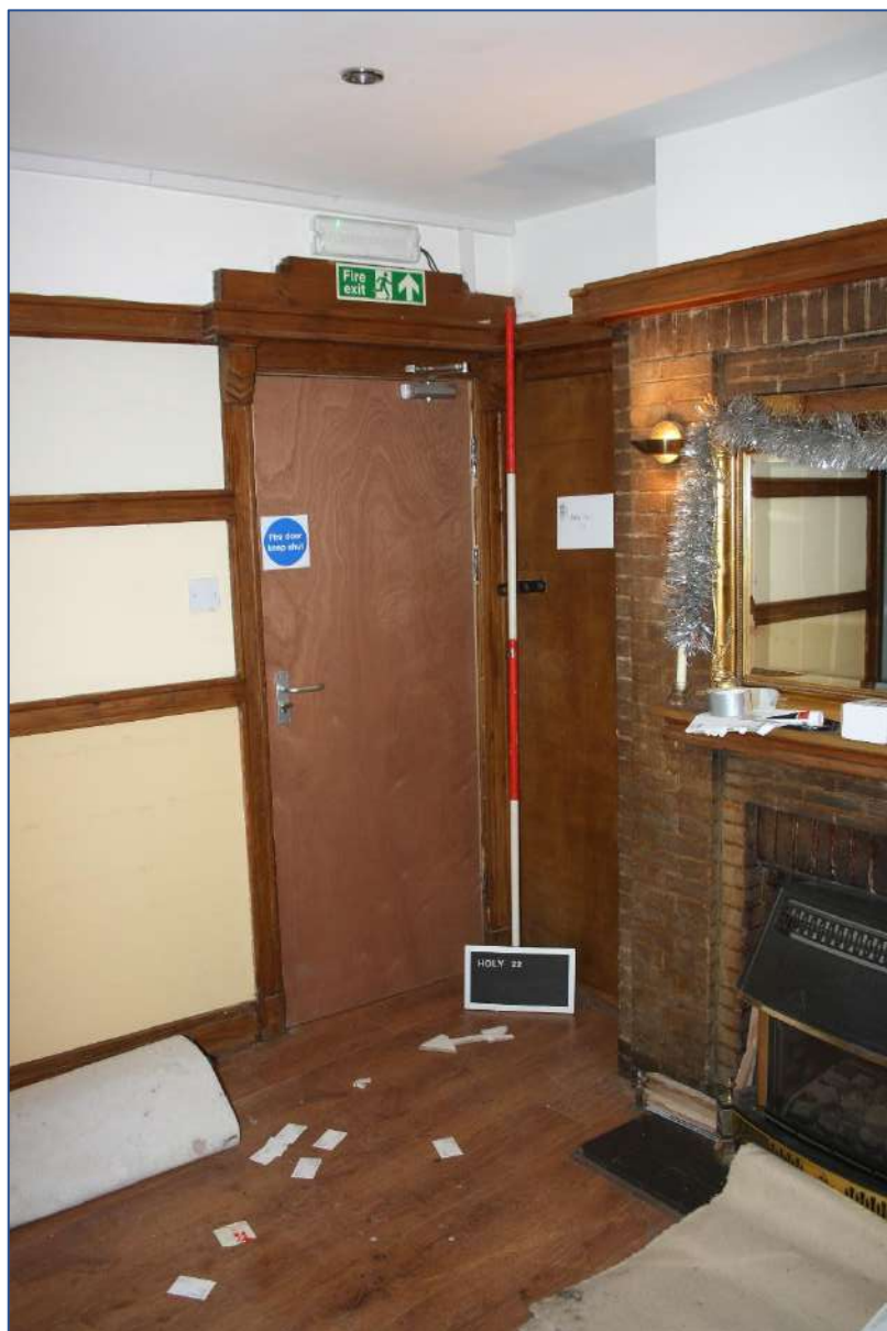
Plate 27: Room 6 looking E.
