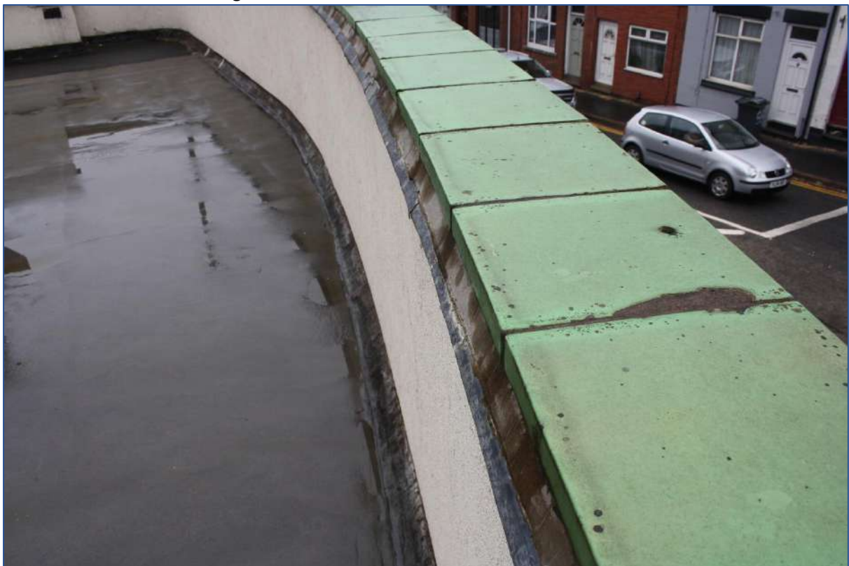
Plate 69: Roof area 27 looking at tile detail, looking W.
