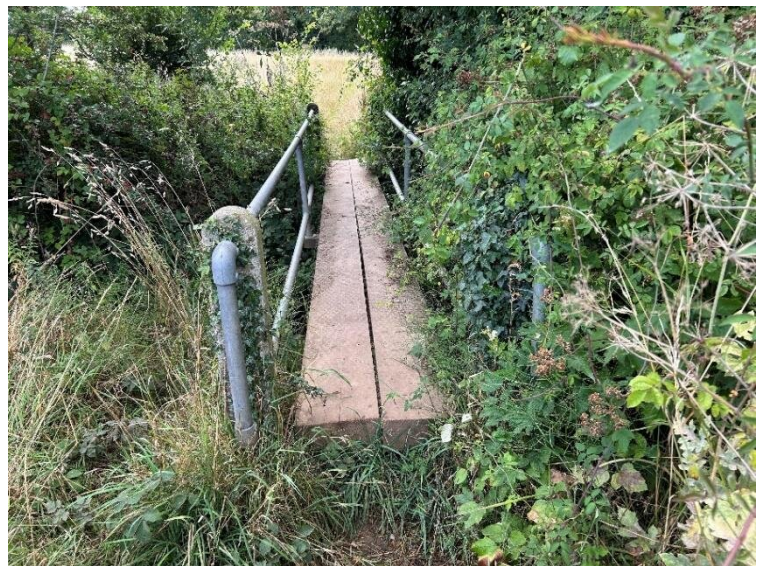
Picture 20 – View of footbridge to the south of the site crossing over stream.
