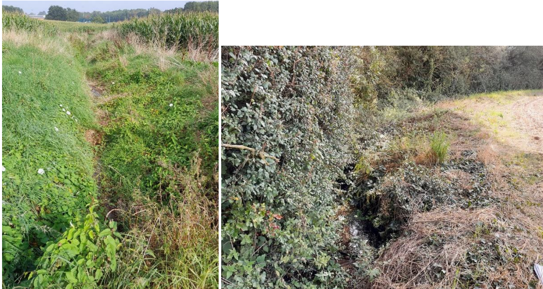
Photograph 2 & 3: Watercourse – WC1 (left), WC2 (right)
