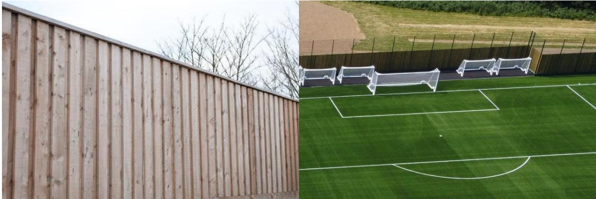
Figure 8 - A Typical Example of an Acoustic Fence
