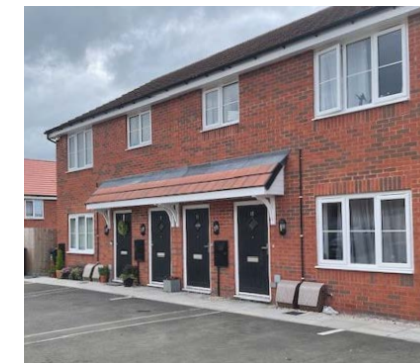
More recent interpretation of terraced housing with shared mono pitch door canopies.
