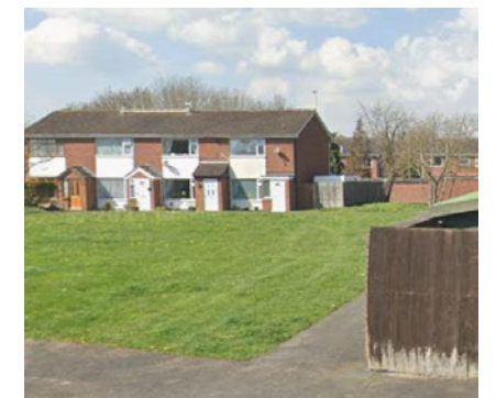
Buildings fronting onto area of greenspace off Cunners Close.
