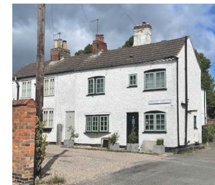
Prominent chimneys on key buildings.
