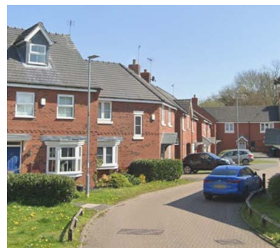
Variations in roof height and styles create interesting roofscape, adding character.
