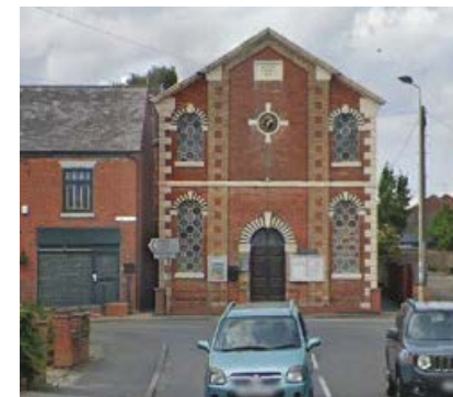
Taller building at key node within village centre, creating a focal point and terminating vista.
