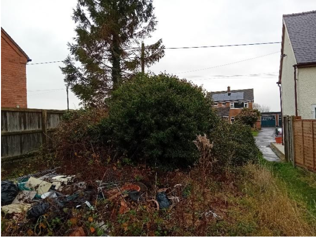
Photo 13: South elevation of building B3, covered in bramble and ivy.
