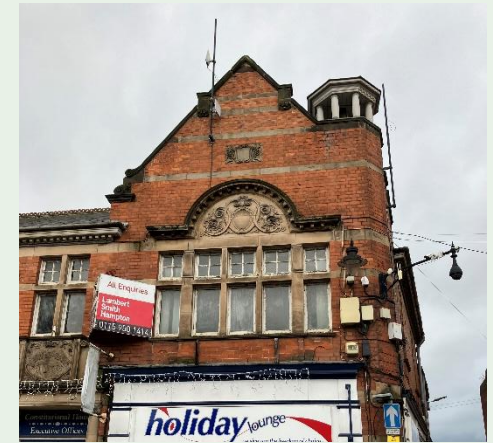
Domed corner rooftop pavilion at 8 Station Rd, Hinckley
