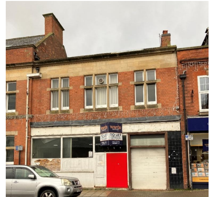
The post office counter shopfront now
