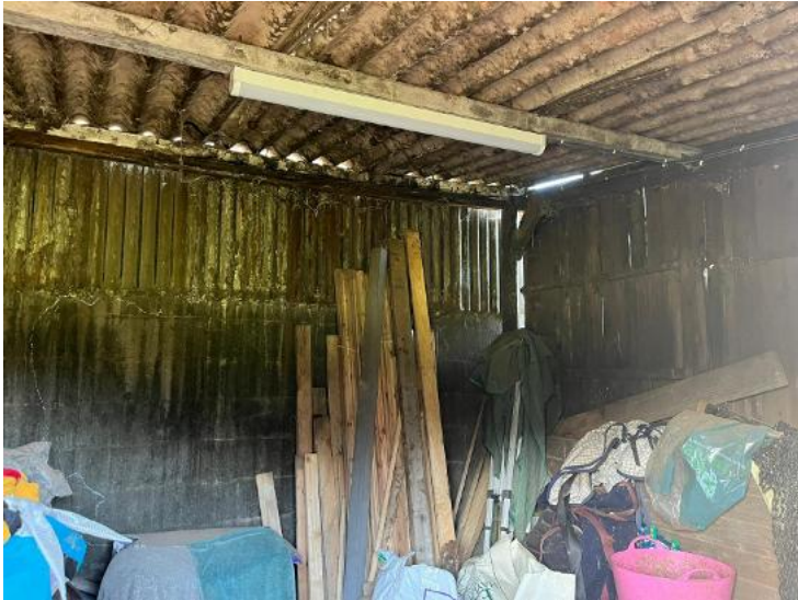
Photo 13: B1 lean-to interior
