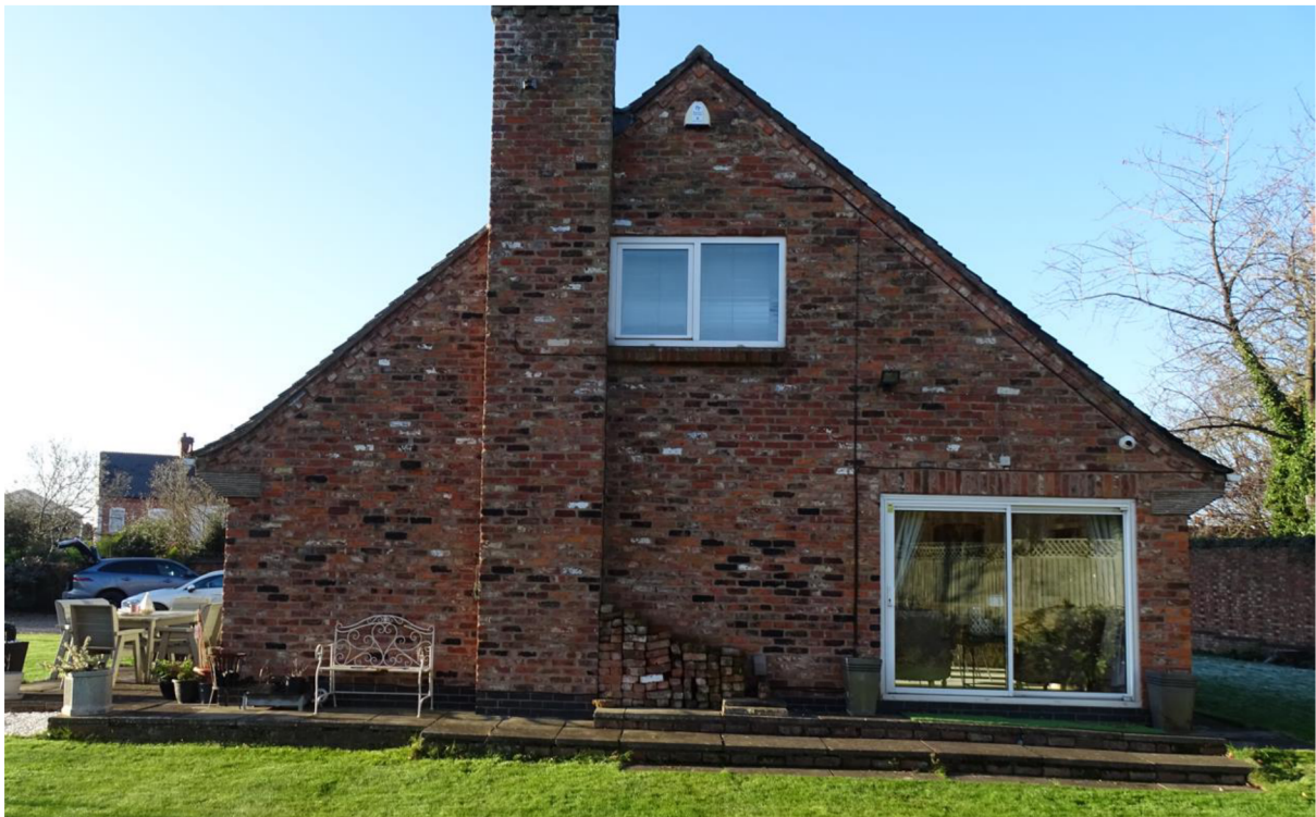
Image 3 – East facing elevation of the property
