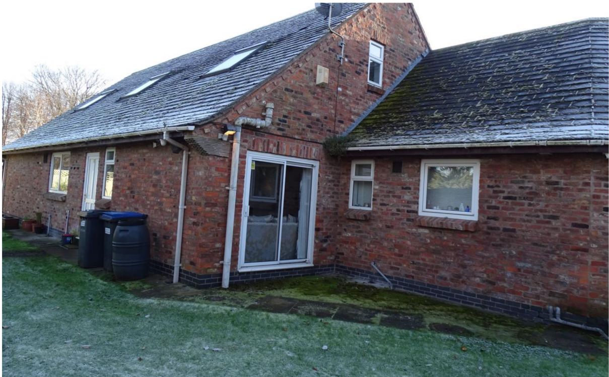
Image 5 – North facing elevation of the property
