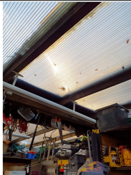
Photo 10: Inside of garage – clear roof panels
