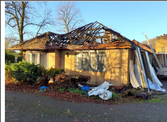
Photo 1: Bungalow taken from southern corner
