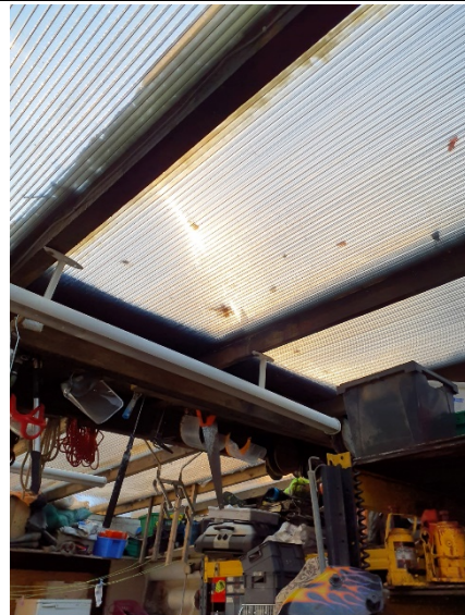
Photo 10: Inside of garage – clear roof panels
