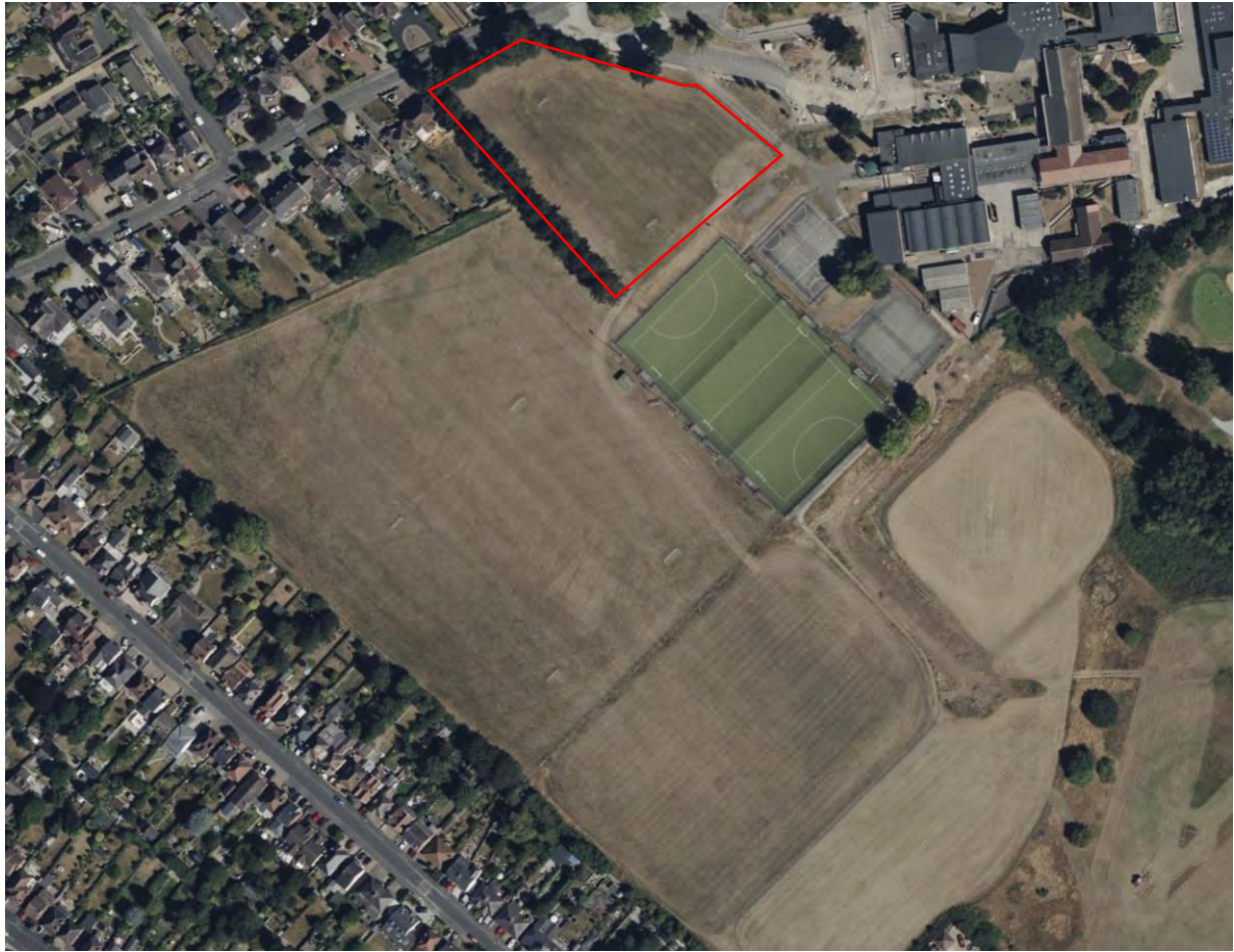
Figure 2: Aerial Image during drought conditions showing discoloured angled lines at the surface as evidence of herringbone field drainage to playing fields. The area of temporary accommodation exhibits no evidence of any existing field drains from records, anecdotal or aerial imagery.
