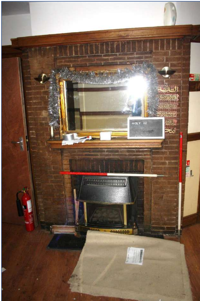
Plate 29: Room 6 looking S/E.
