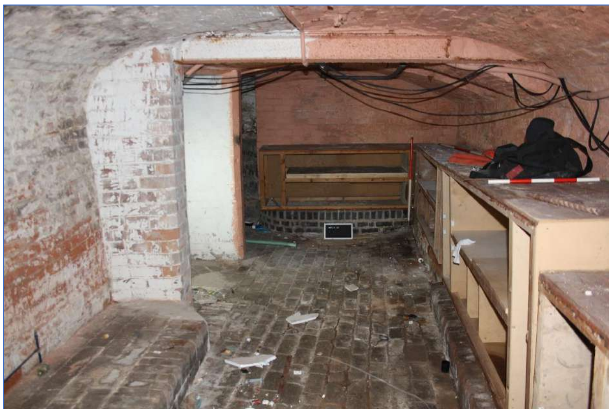
Plate 81: Brick vaulted Cellar A looking north.
