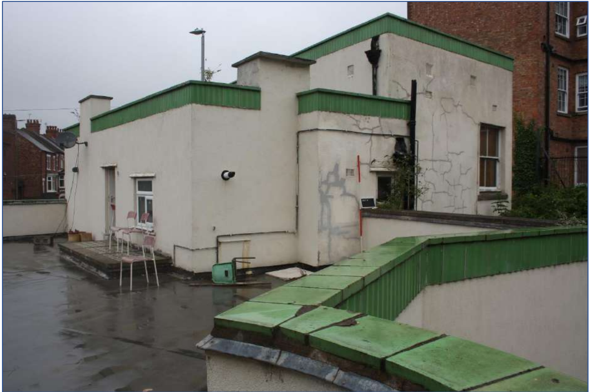
Plate 72: Roof area 27 looking N.
