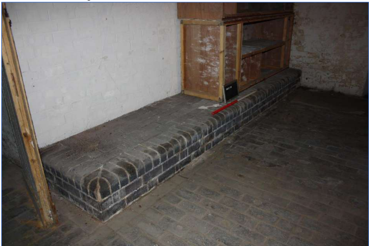
Plate 86: Brick Thrawl in Cellar B looking southeast.
