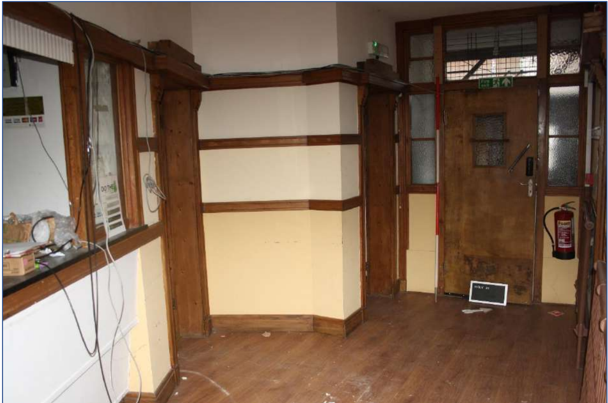
Plate 23: Room 5 Entrance Hall looking N/W.
