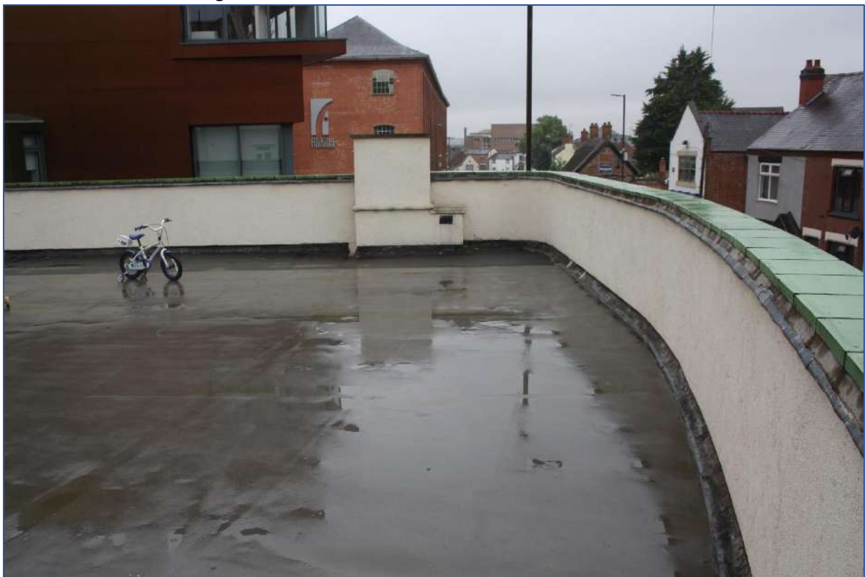
Plate 67: Roof area 27 looking S/W.
