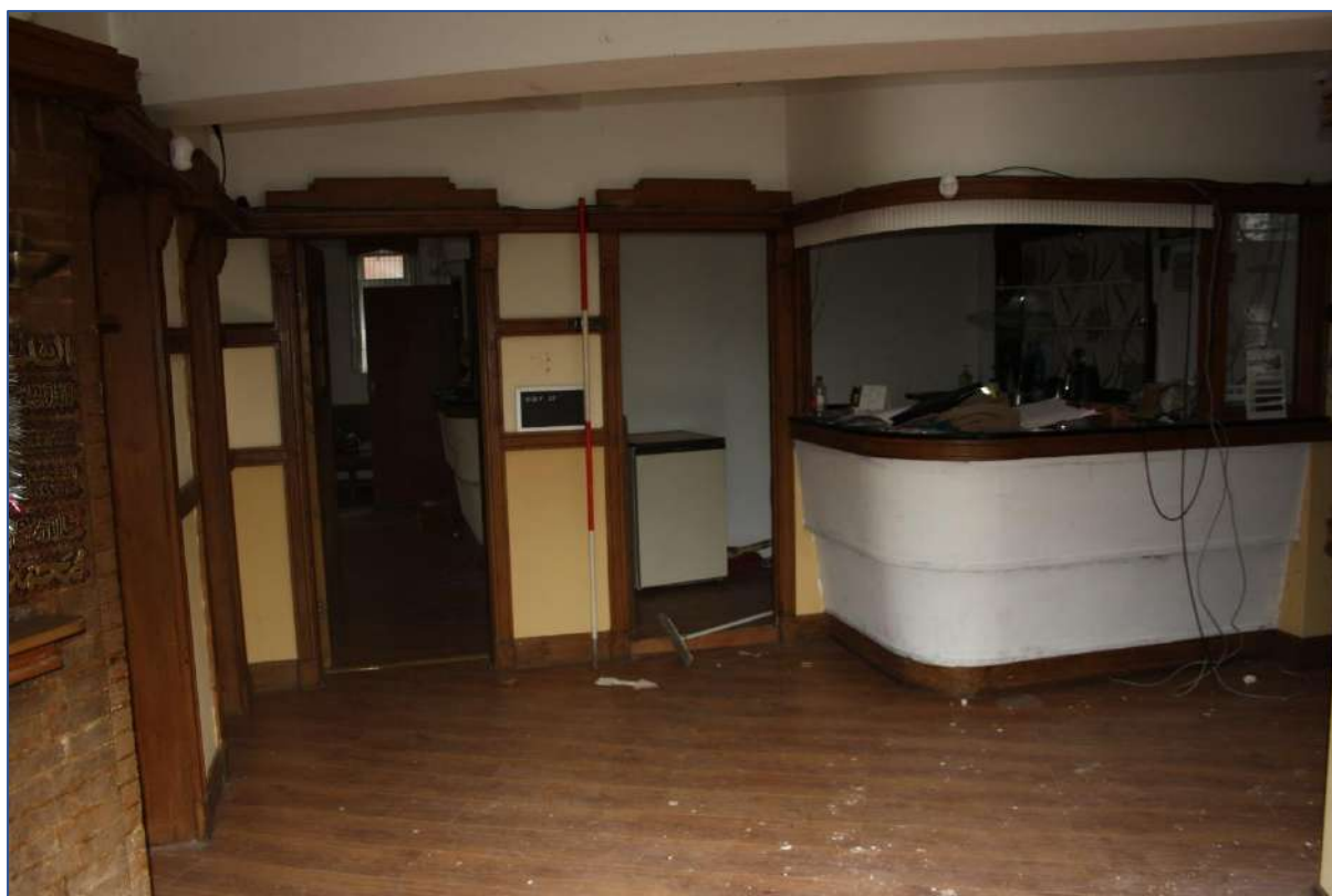
Plate 28: Room 6 looking S/W towards Room 5.
