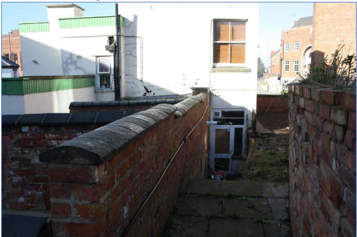
Plate 5: Rear entrance looking N.
