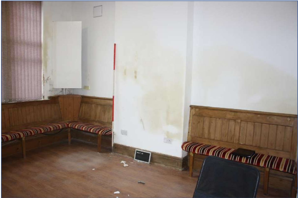
Plate 47: Room 3 looking E.
