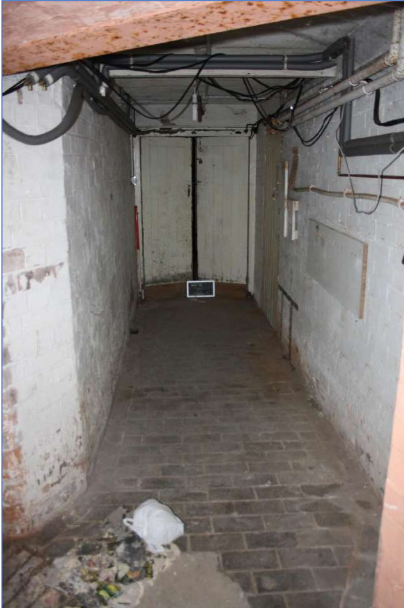
Plate 78: Cellar Corridor looking southwest.
