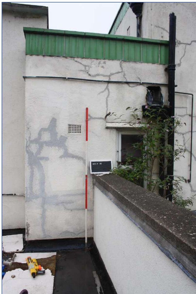
Plate 73: Roof area 27 looking N/W.
