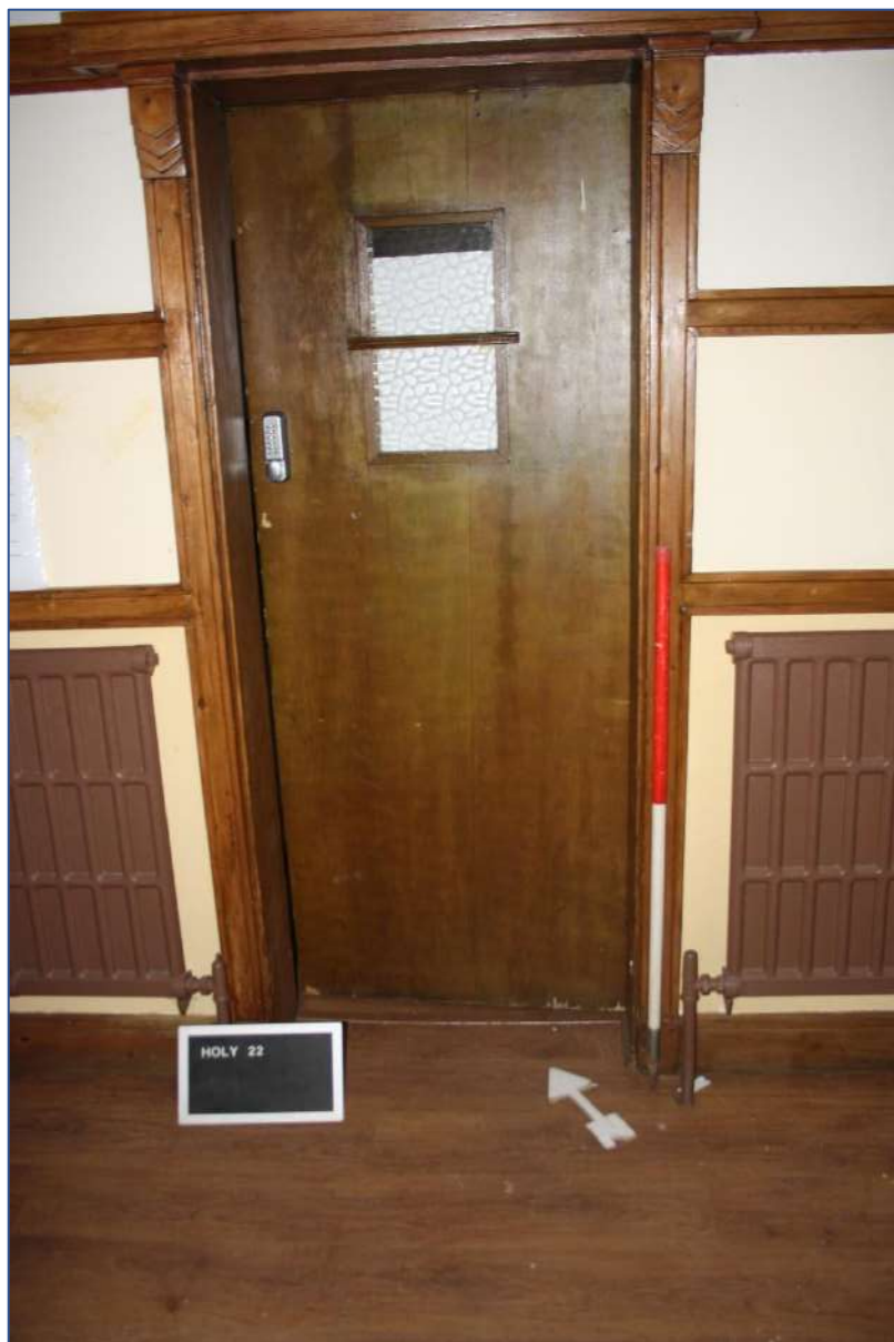
Plate 51: Room 5 looking E to door leading to 2.
