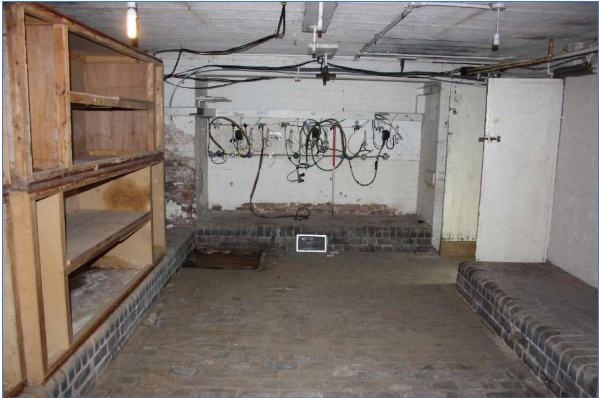
Plate 87: Cellar B looking northwest.
