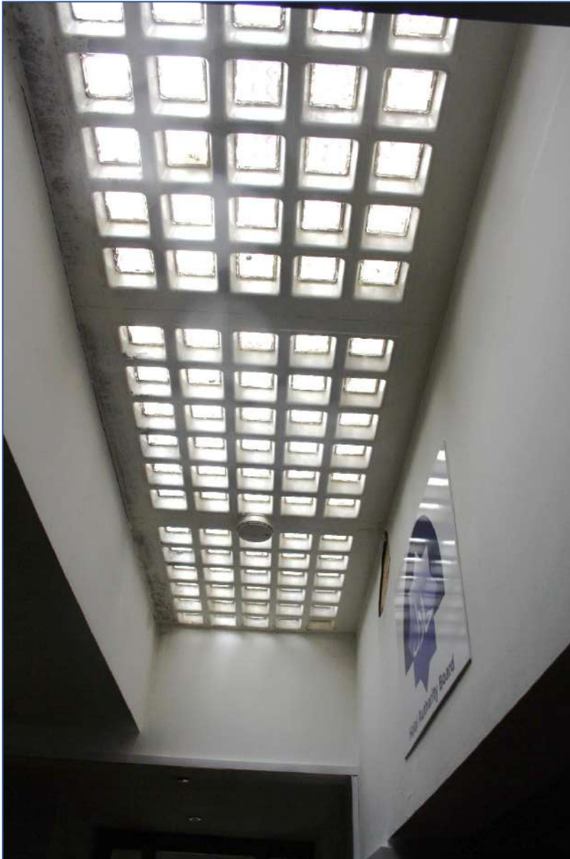
Plate 30: Room 5 ceiling looking N/W.
