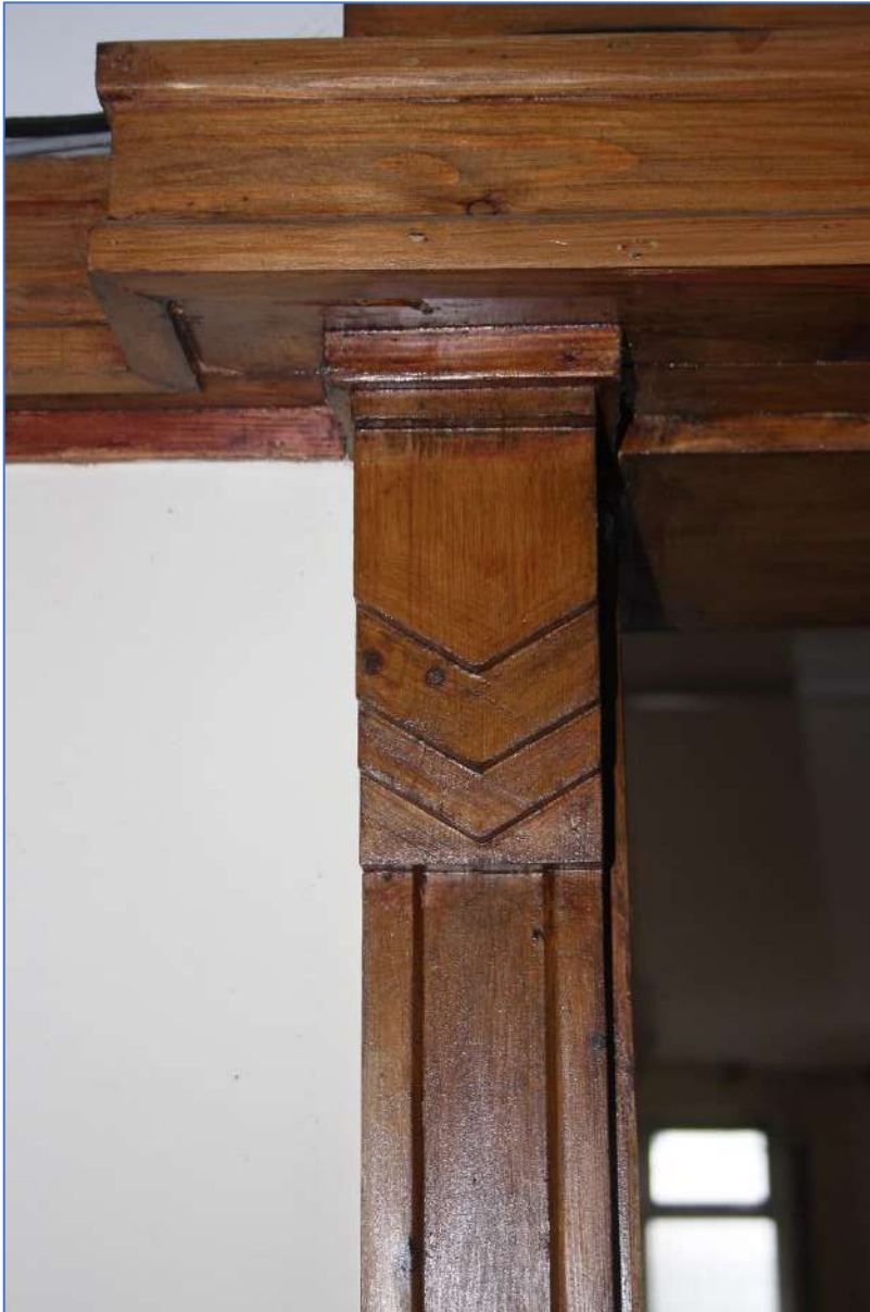
Plate 8: Door frame detail looking N/E.
