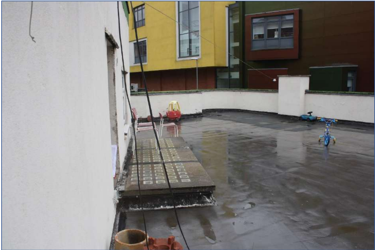
Plate 70: Roof area 27 looking S/E.
