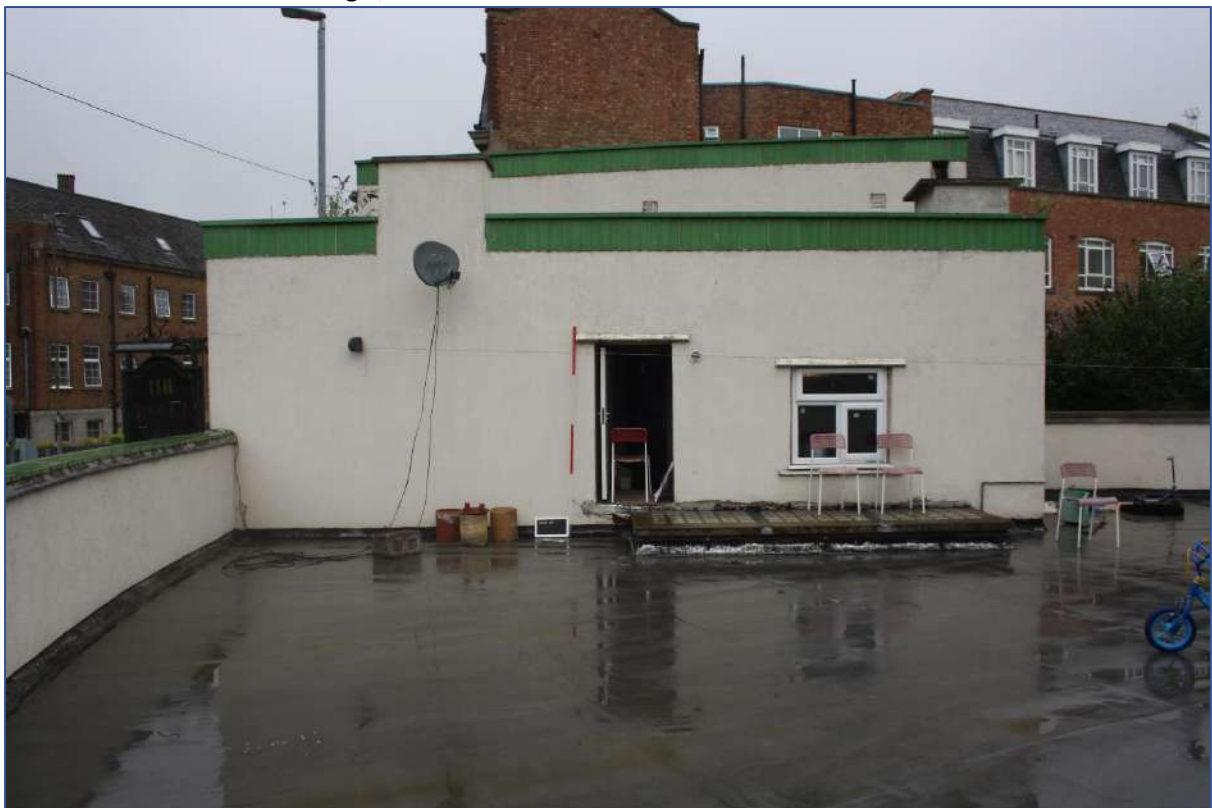
Plate 71: Roof area 27 looking N/E.
