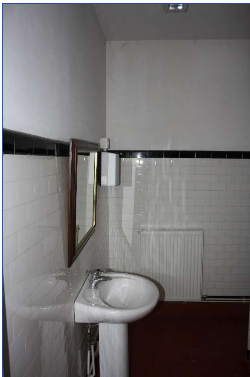
Plate 32: Room 11 looking N/W.
