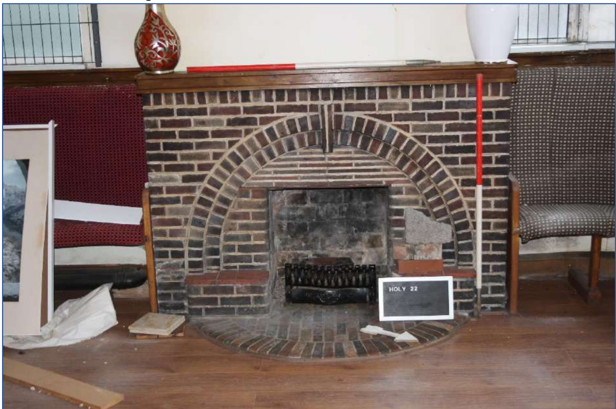
Plate 19: Room 1 fireplace detail looking S/W.
