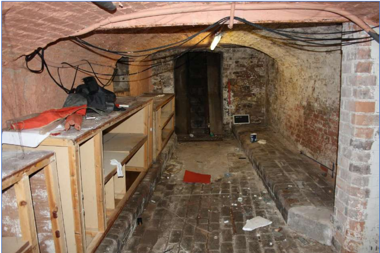
Plate 76: Vaulted brick Cellar A looking south.
