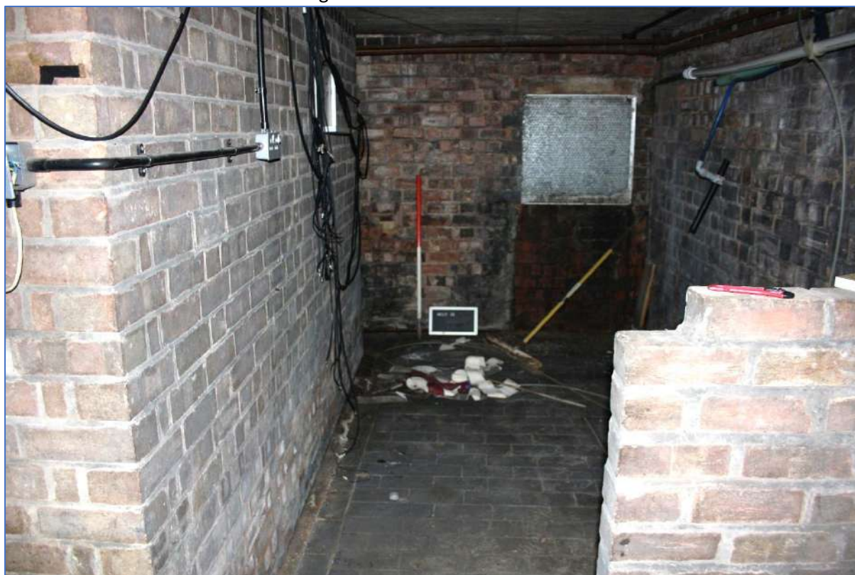
Plate 82: Cellar C looking southwest.
