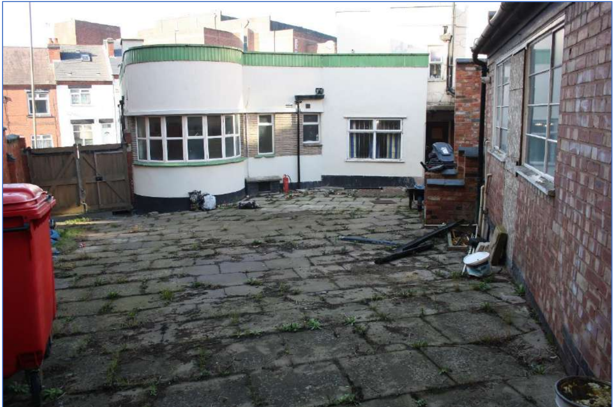
Plate 4: Elevation CC looking N/W.
