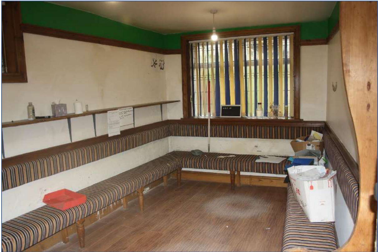
Plate 41: Room 10 looking S/E.
