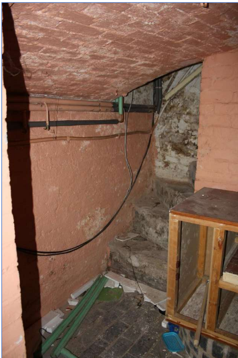
Plate 75: Cellar A steps leading up.
