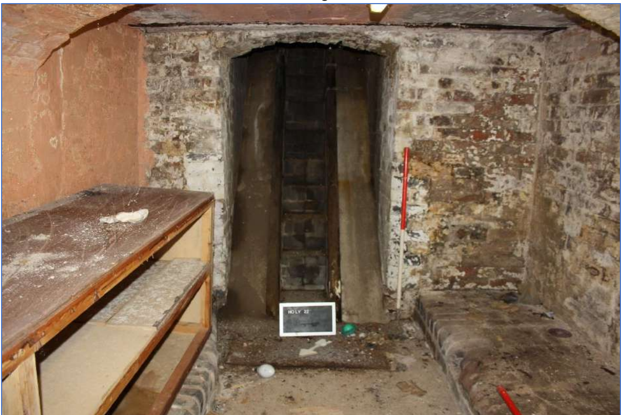
Plate 80: Barre Roll Roll looking south in Cellar A.
