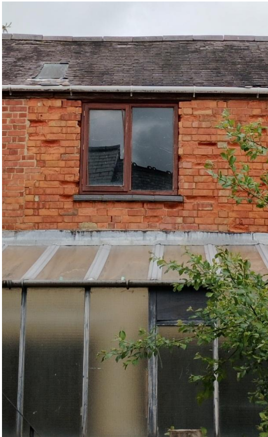
Photograph 6: Rear elevation showing windows and roofline.
