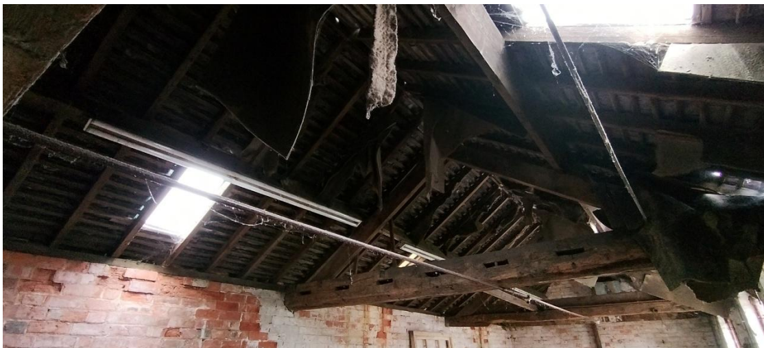
Photograph 2: Internal roof space showing exposed timbers and open roof void.
