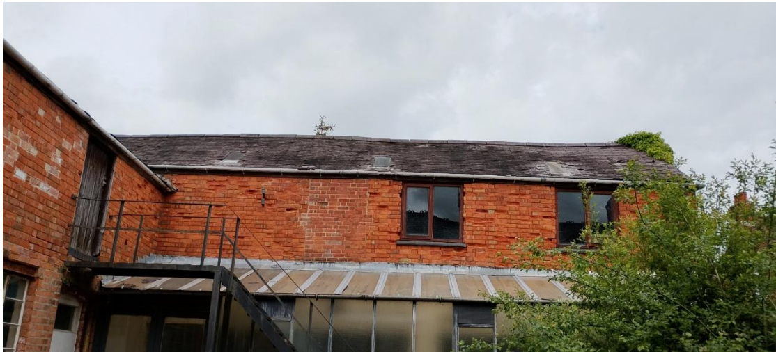
Photograph 8: Rear elevation showing roof slopes and surrounding vegetation.
