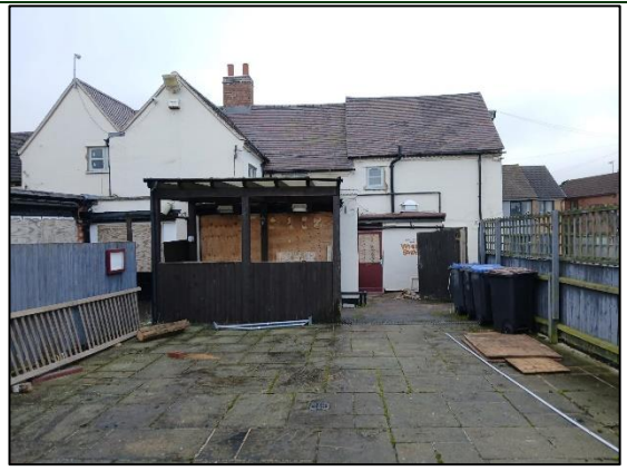
Photograph 4: building(s) to the east of the Site
