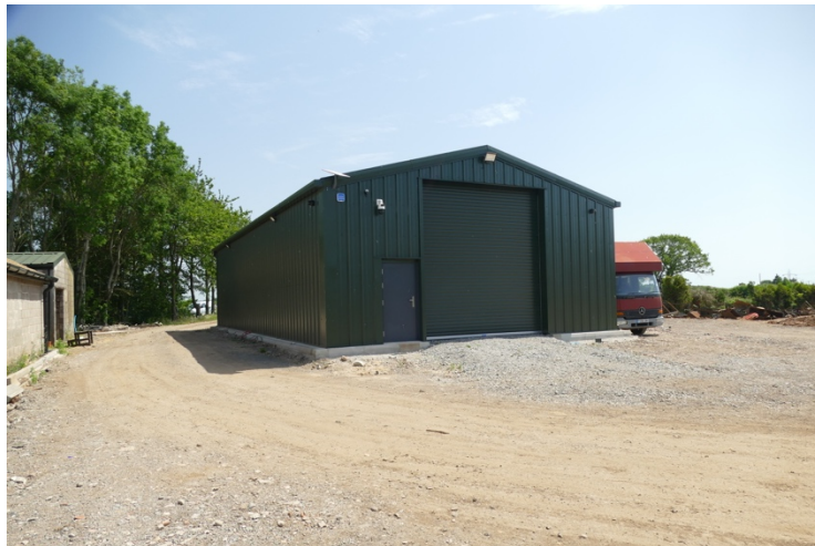
Photograph 3 – Farm track and buildings Pond 4 and development site
