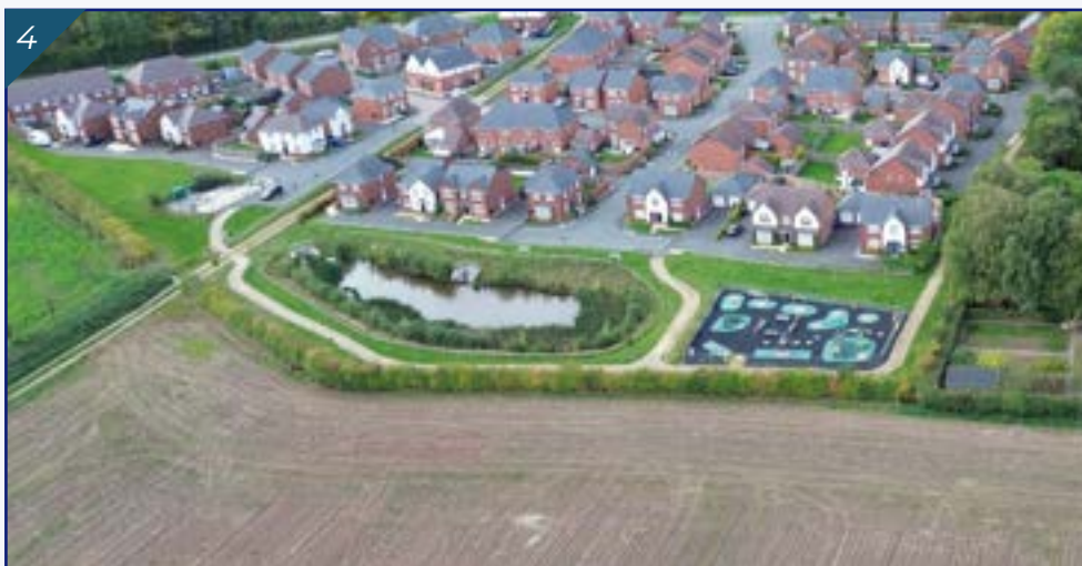
View toward the play area and attenuation basin adjacent to the western boundary of the site.
