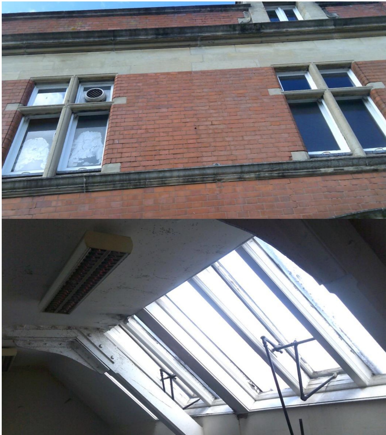
Internal 3 rd storey showing small loft (inaccessible)
