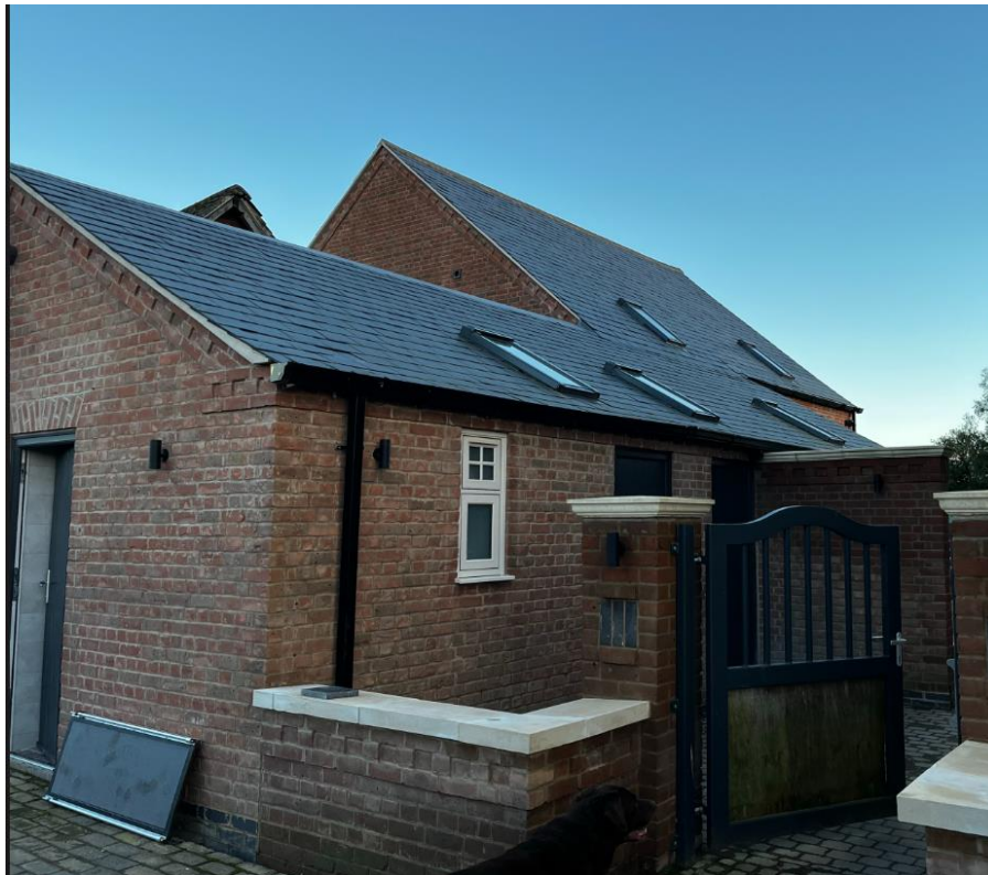
Photo 3 – Replacement Ancillary Building (Building B)
