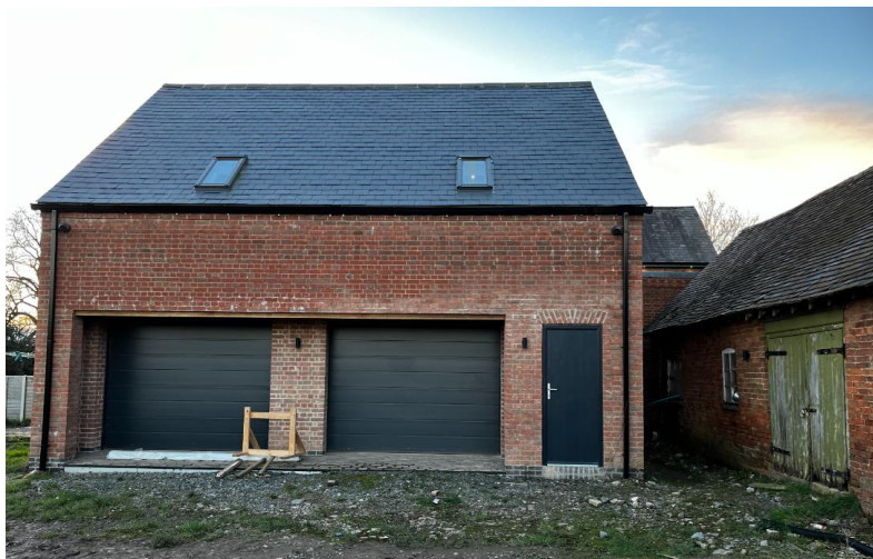
Photo 4 – Double Garage (Building A)
