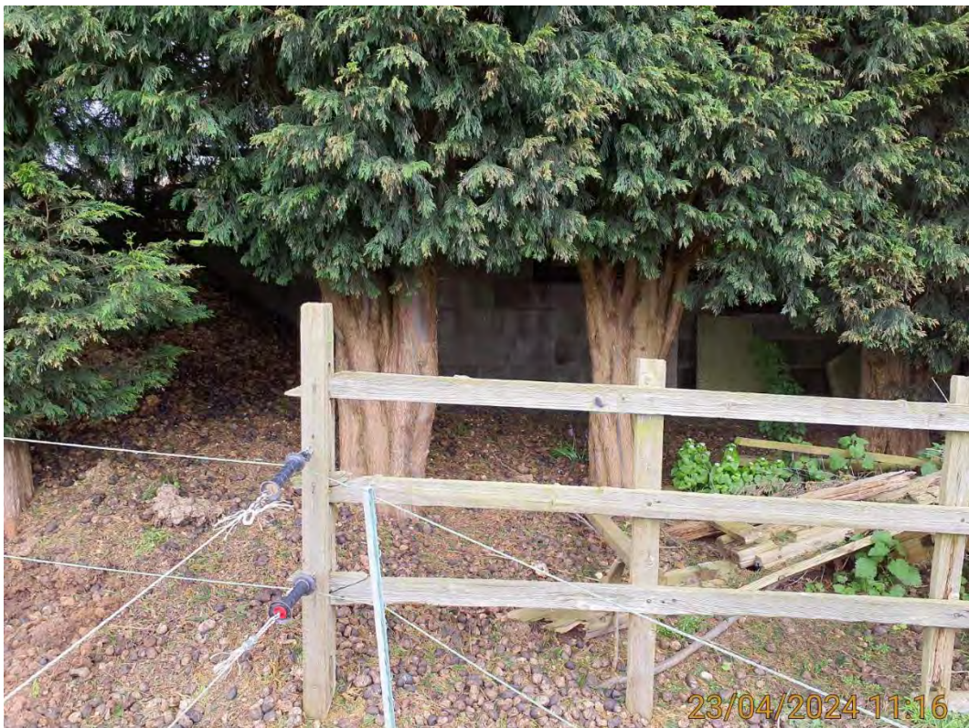
Plate 10 – View south of the retaining wall in the southwest of the site
