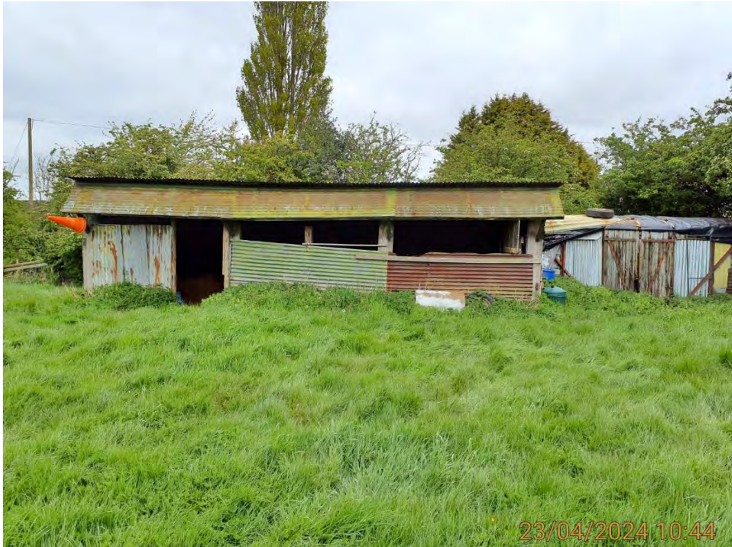
Plate 11 – Animal shelter and storage building in the northeast corner of the site
