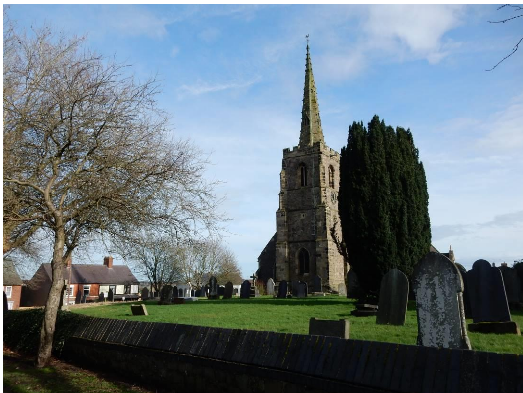
Plate 15: West tower of Grade II* listed Church of St Simon and Jude
