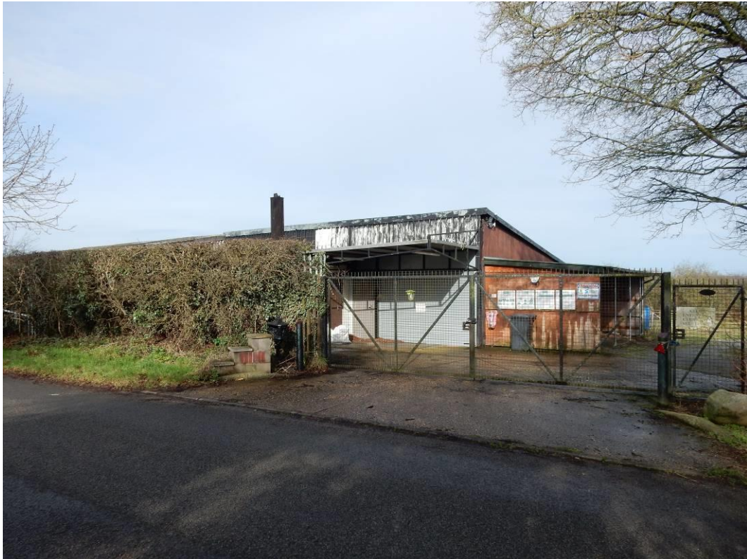
Plate 9: Building on north side of unnamed road, north of application site
