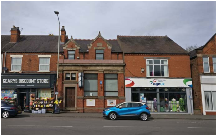
EARL SHILTON HIGH STREET - CONTINUOUS FRONTAGE
