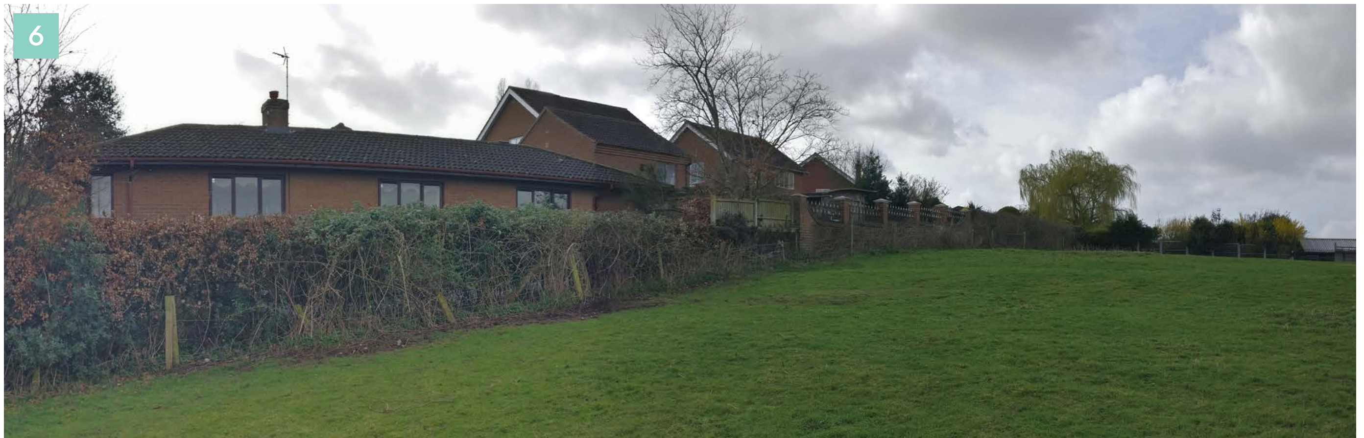
VIEW OF SOUTHERN BOUNDARY SHARED WITH DWELLINGS OF CLEAR VIEW CRESCENT
