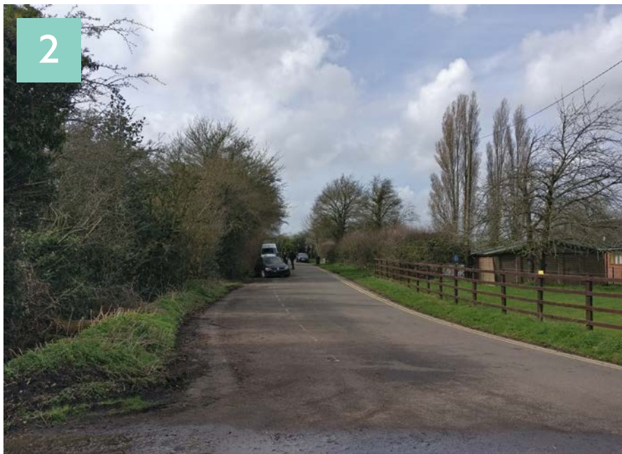
VIEW WEST ALONG UN-NAMED ROAD
