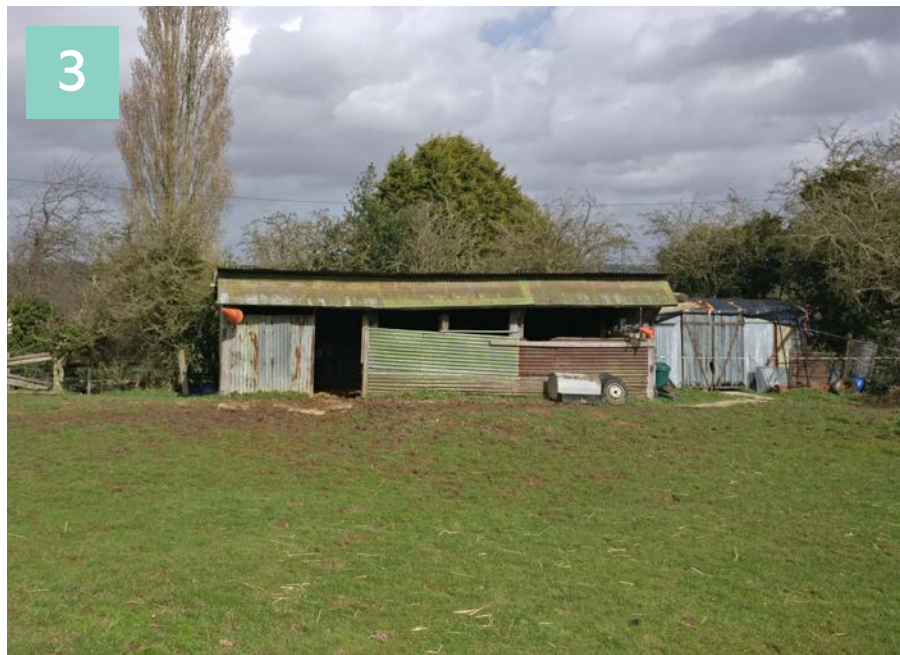
EXISTING STABLES BUILDING IN NORTHEAST CORNER
