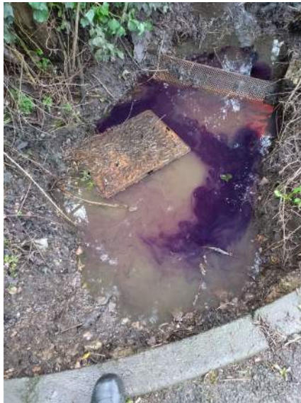
Ditch water dye goes to MH cover edge iii.JPG
