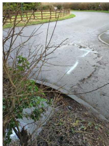
Line from MH blocked ii.JPG
