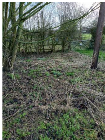
No ditch behind TP.JPG
