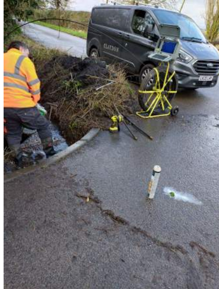
Line from MH traced i.JPG
