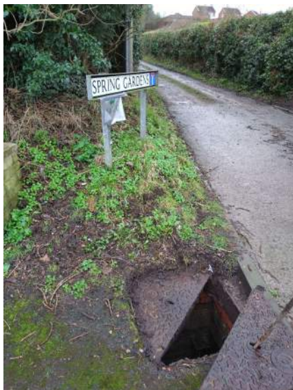
Cables cover opp ditch iii.JPG
