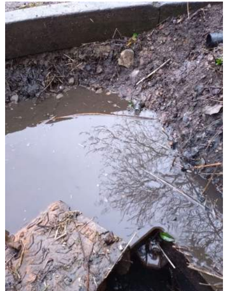
Sm open pipe side of ditch top.JPG
