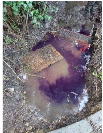
Ditch water dye goes to MH cover edge iv.JPG
