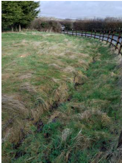
Sm ditch inside NW fence iii.JPG
