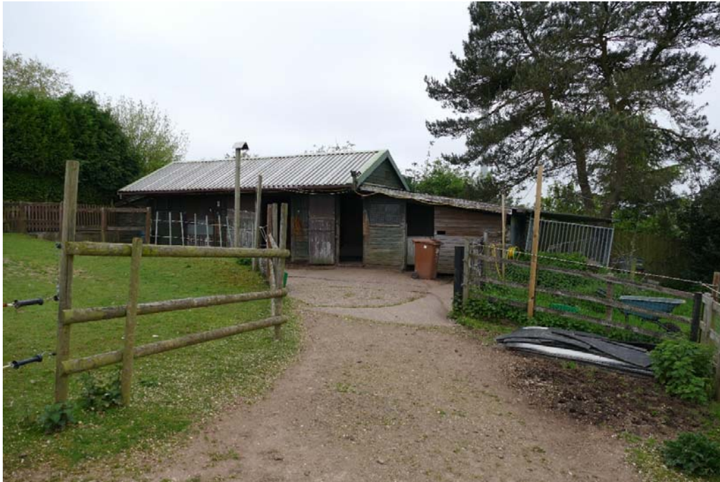
The donkey stables in the south-west corner of the site, looking south-west Fig 19
