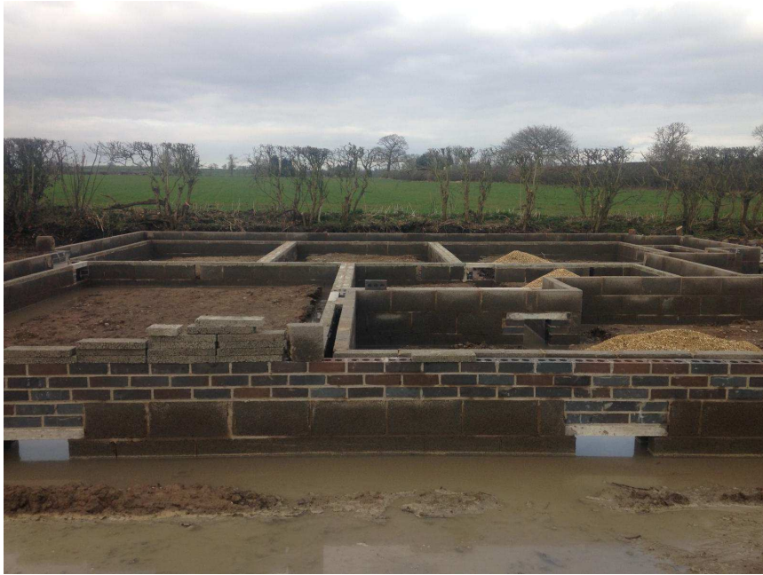
Figure 3 Existing sparse hedge whilst dwelling under construction
