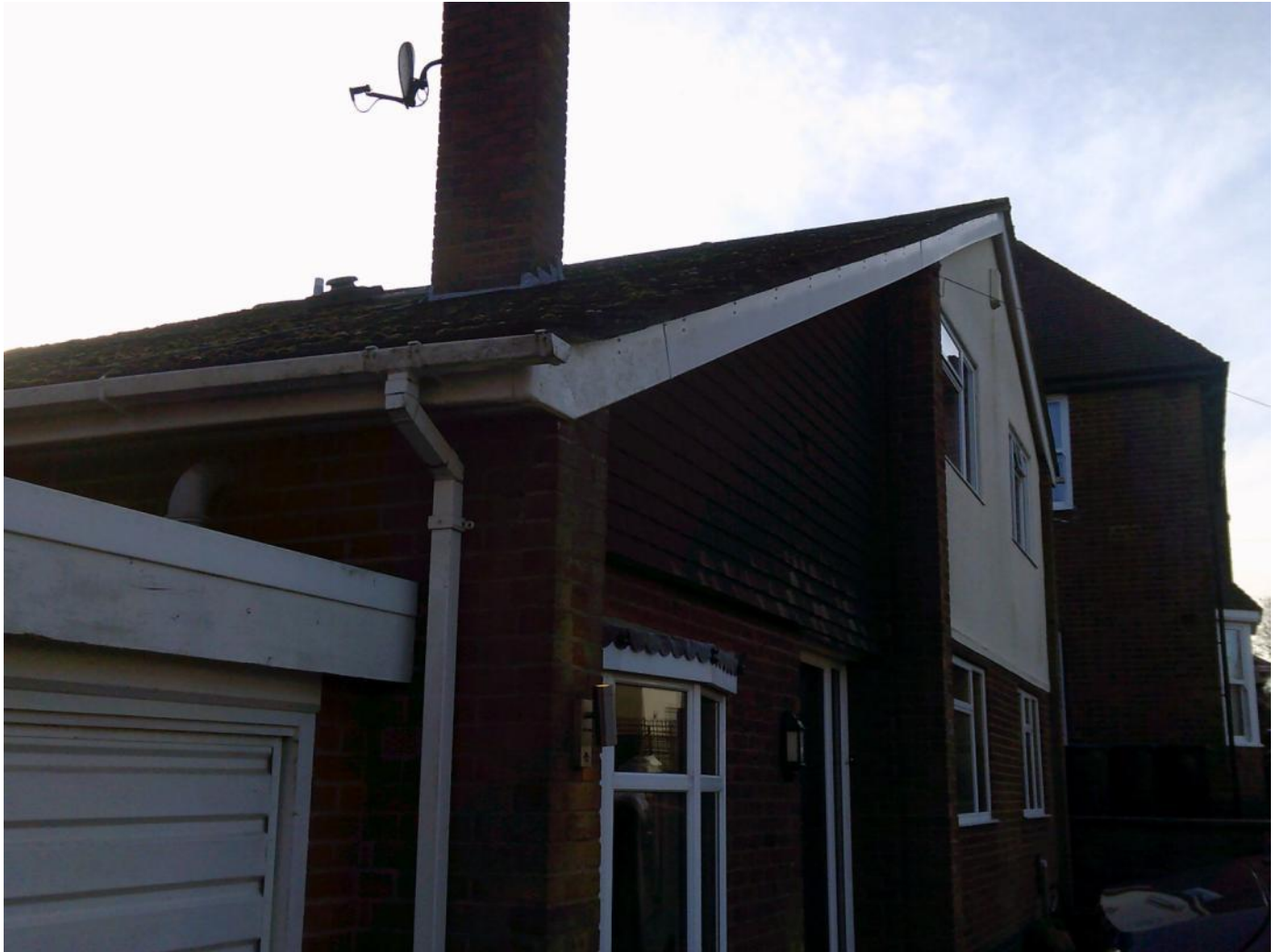
Side elevation flashing intact, tiles intact
