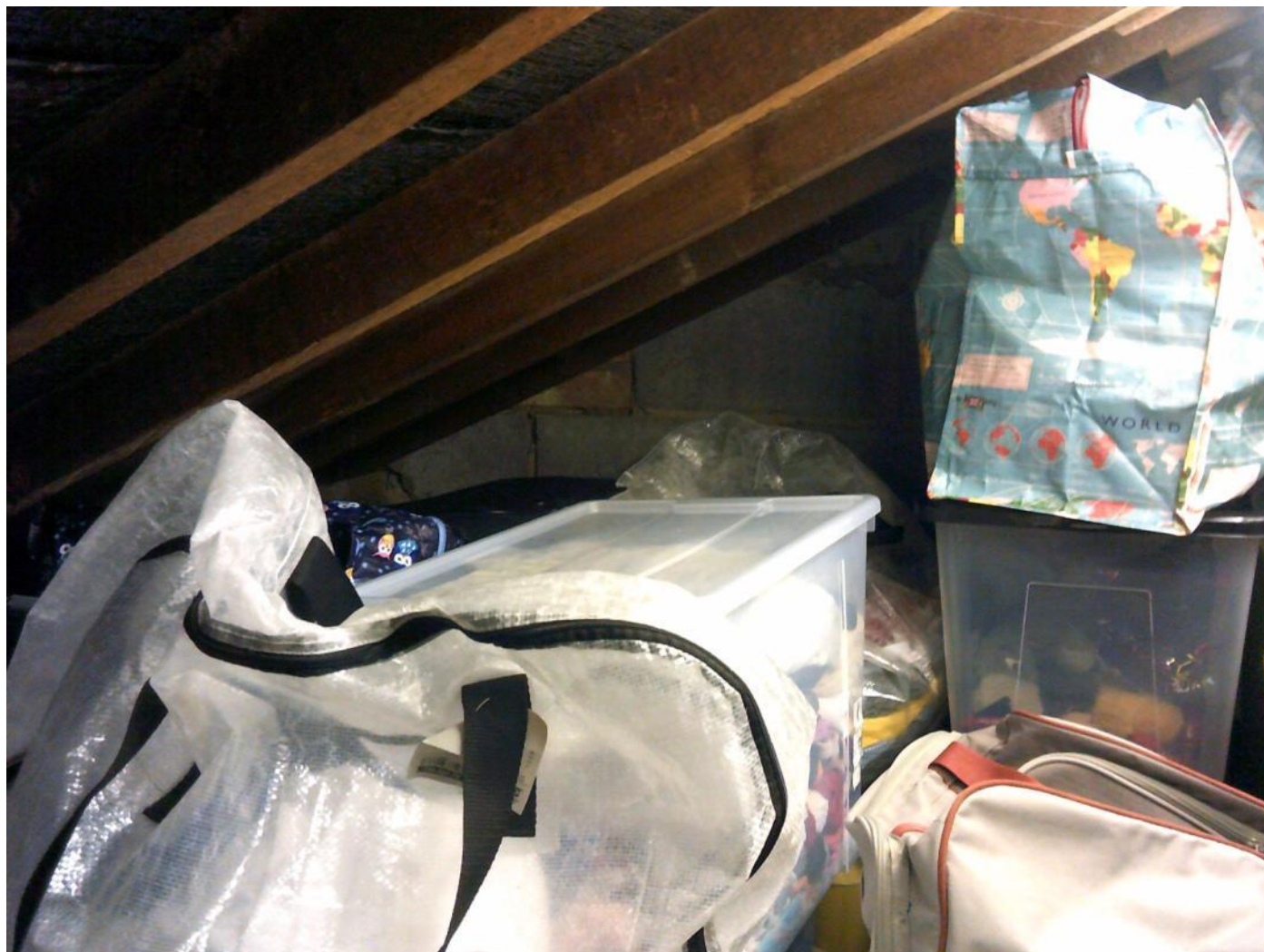
Main roofspace: no evidence bats/birds/vermin
