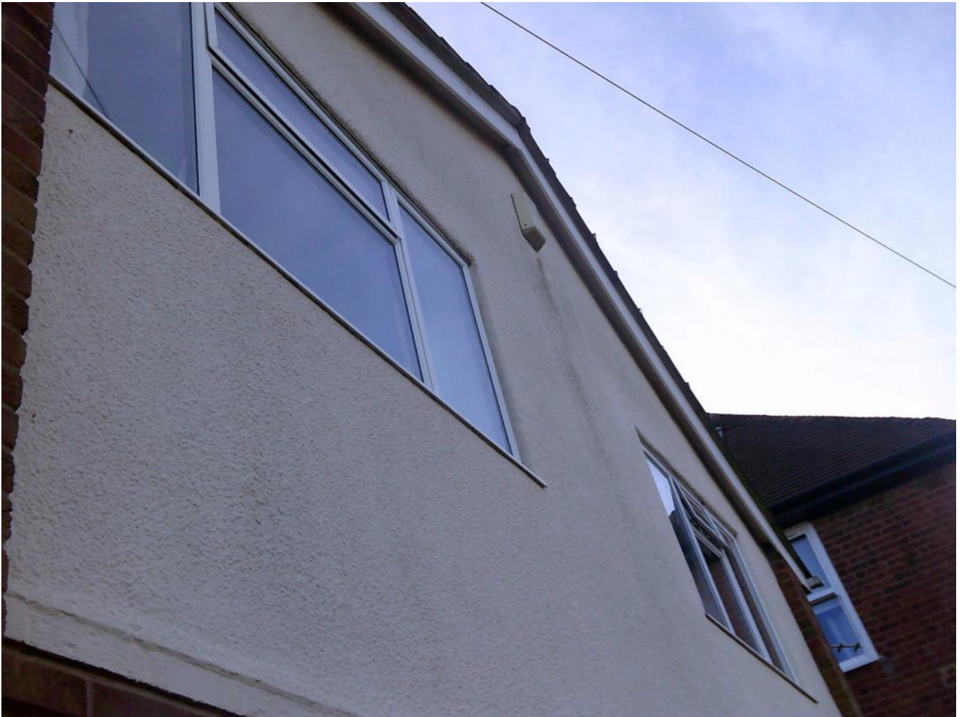
Front elevation intact
