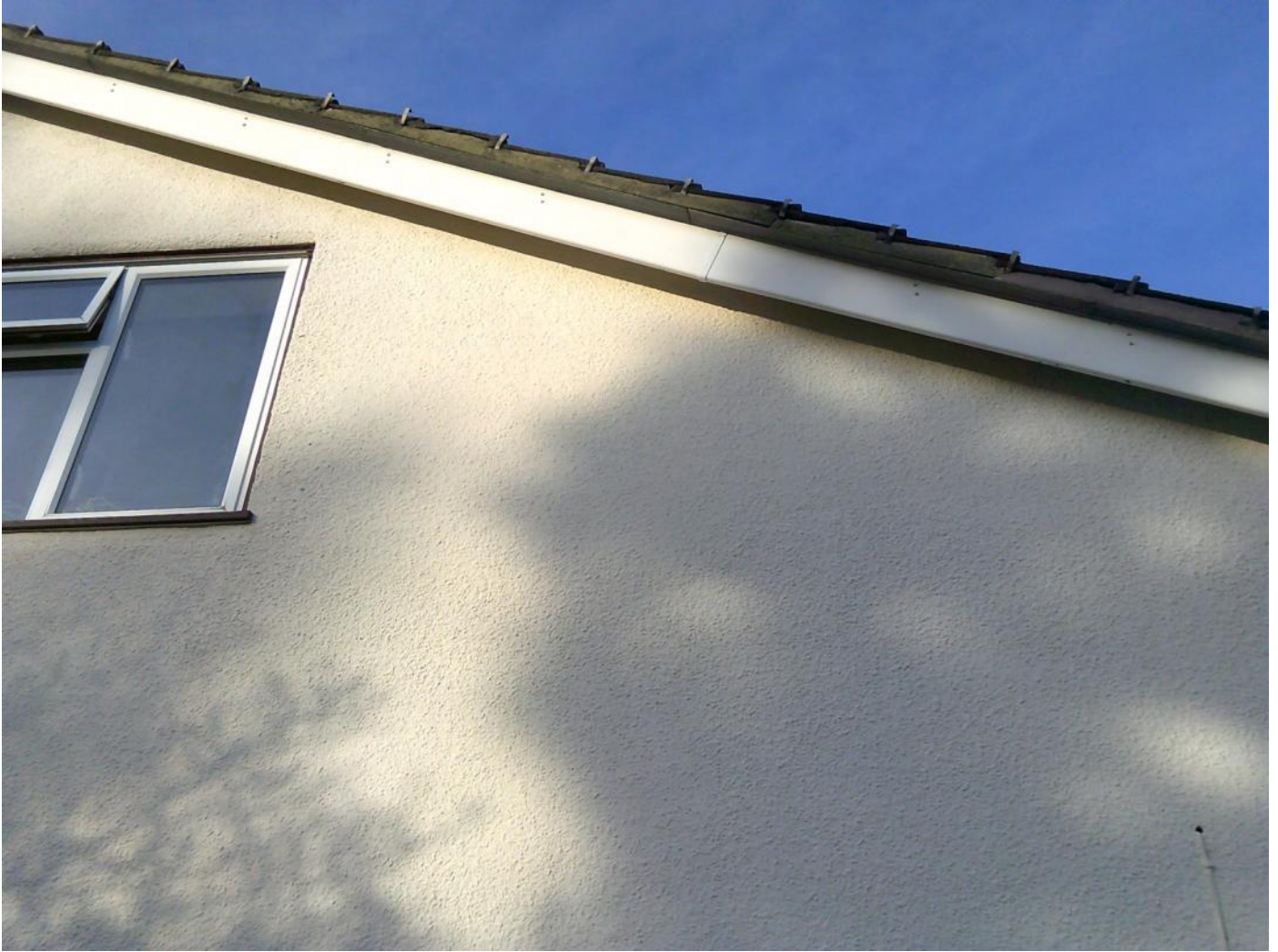
Roof edge mortar intact rear
