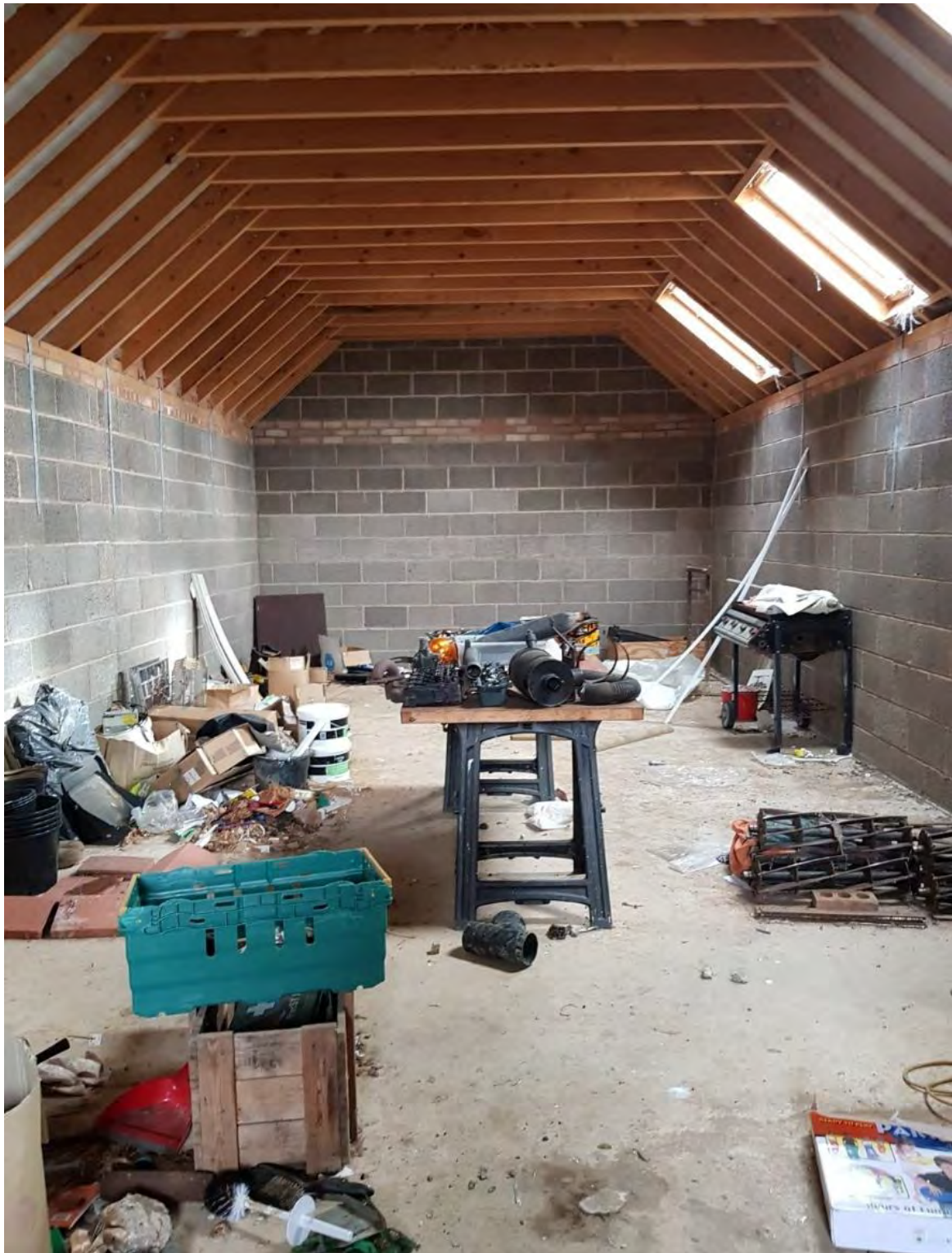
Plate 3: Interior of the new building constructed on the site of Field barn north of Godsons Hill Farm, Market Bosworth (MLE20507)
