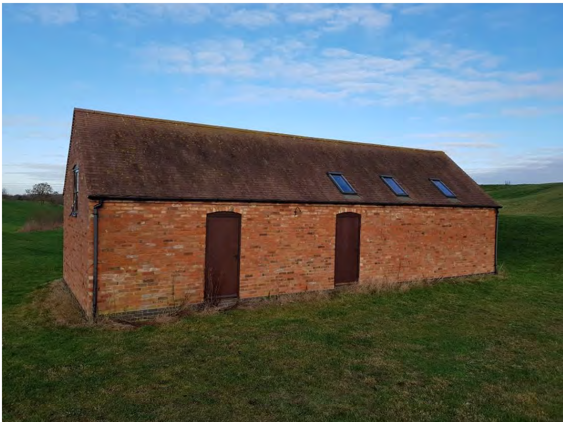
Plate 2: New building constructed on the site of Field barn north of Godsons Hill Farm, Market Bosworth (MLE20507)
