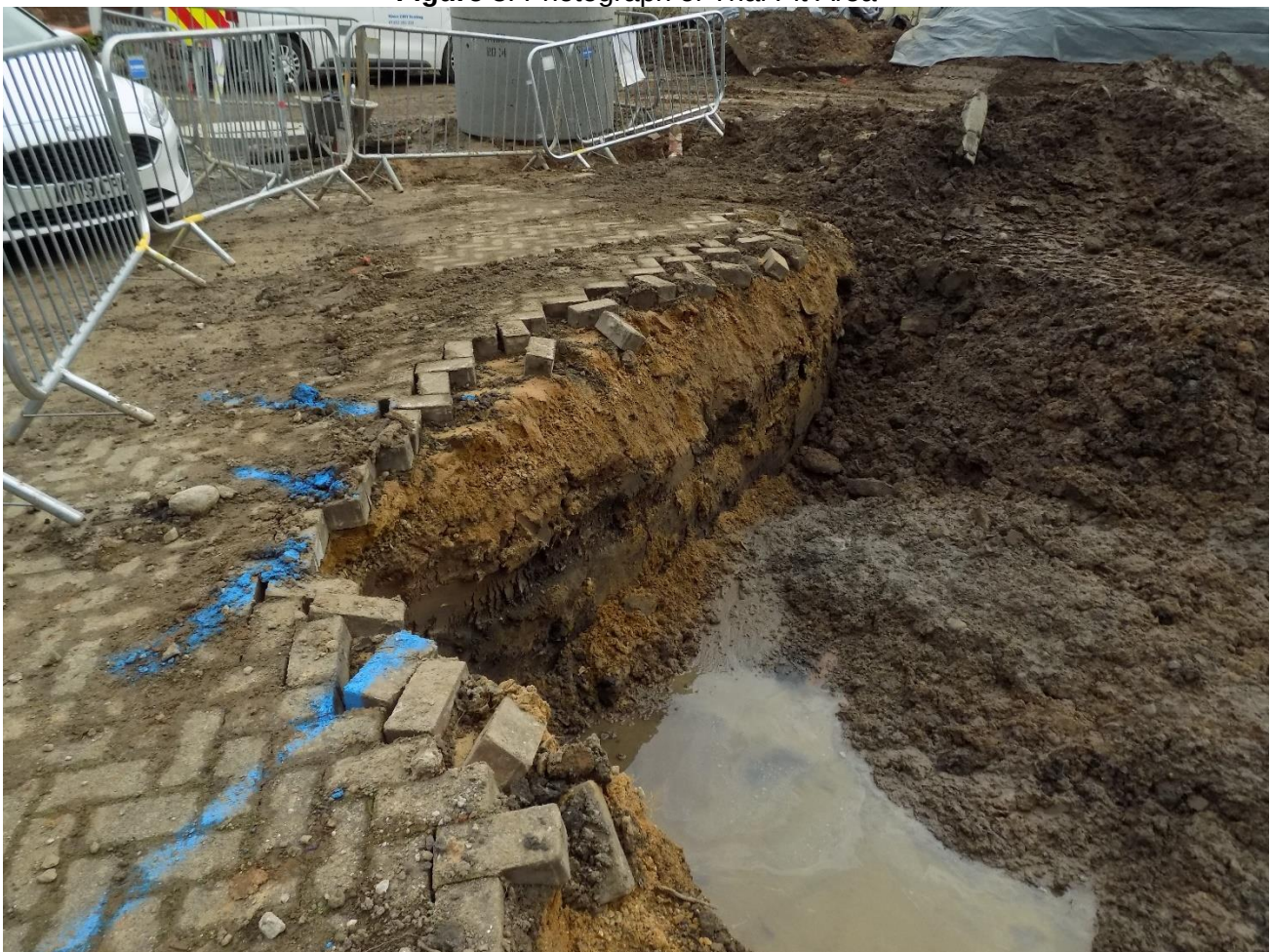
Figure 6: Photograph of Trial Pit Area
