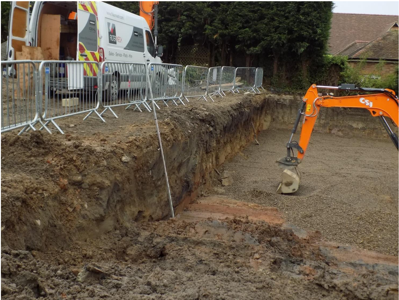
Figure 6: Photograph of Trial Pit Area
