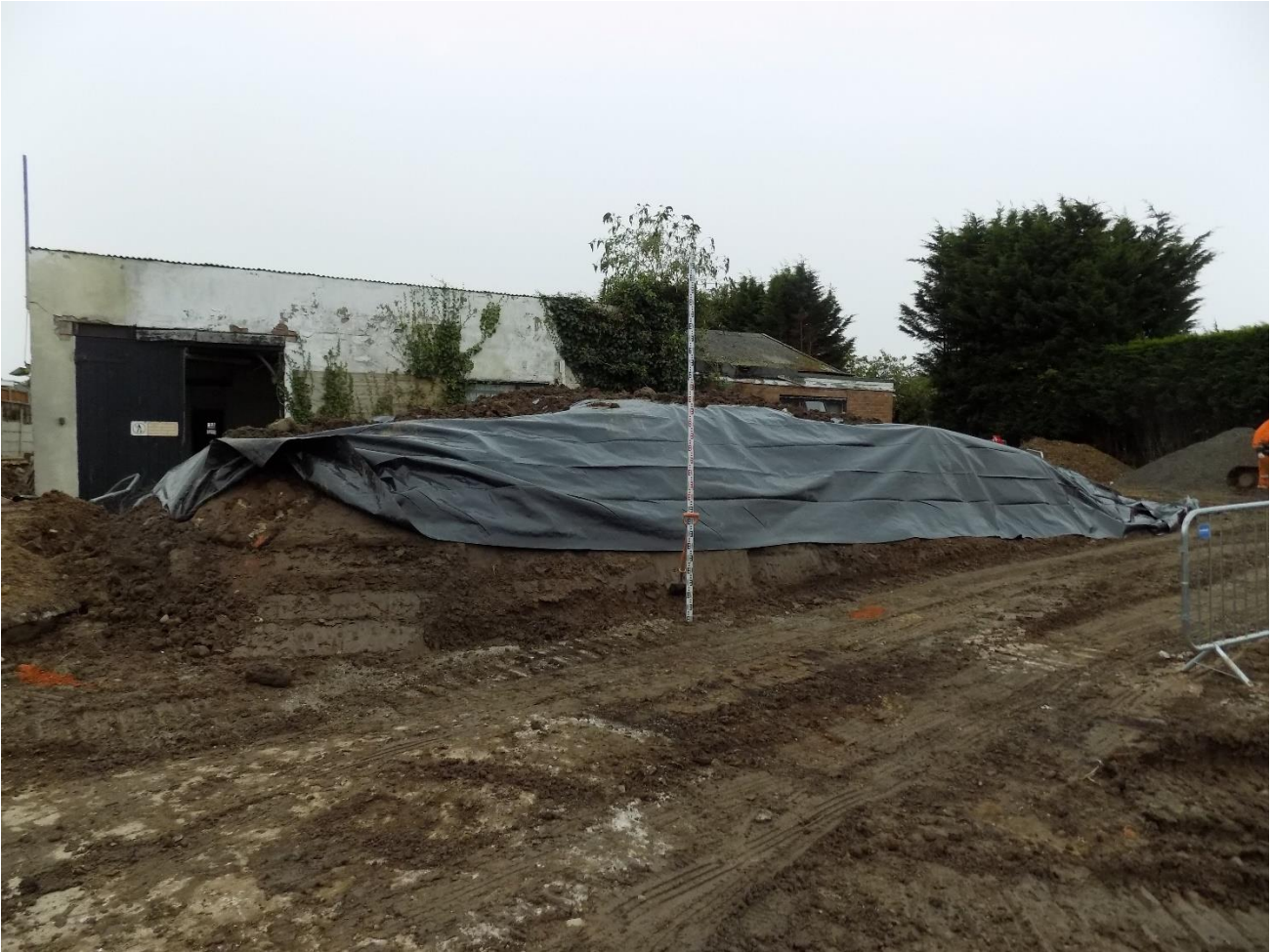
Figure 3: Photograph of Stockpile 2
