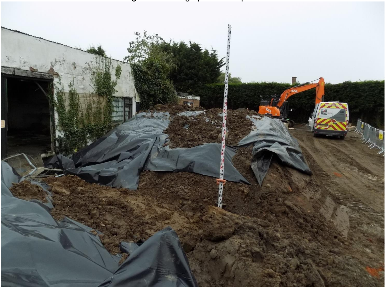
Figure 4: Photograph of Stockpile 2
