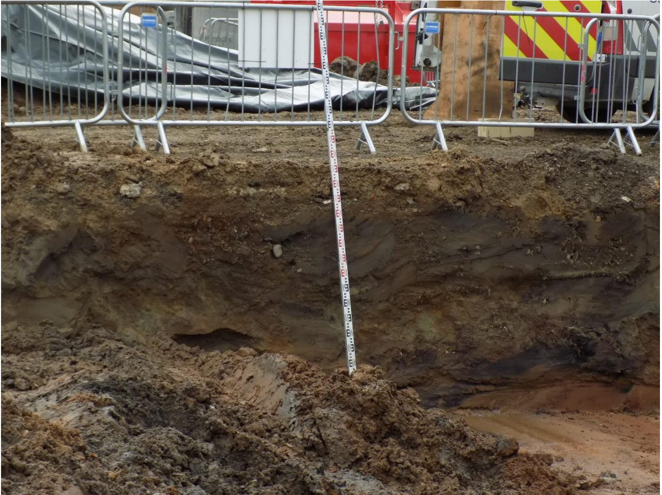
Figure 5: Photograph of Trial Pit Area
