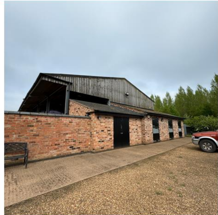
Photo No.2: Facing NW outside the eastern boundary of site showing adjoined units on the eastern face of barn
