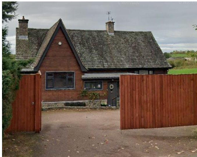
Figure 3 Image of dwelling of similar appearance within the locality.
