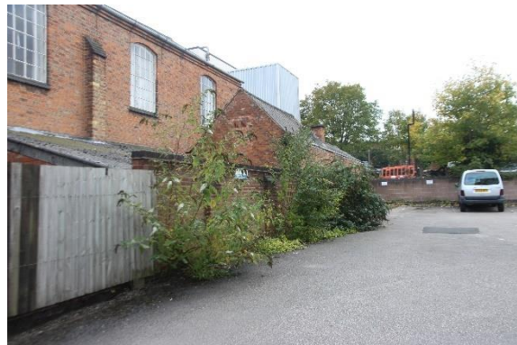
Exterior of storage area showing asbestos cement roof sheeting and timber compound
