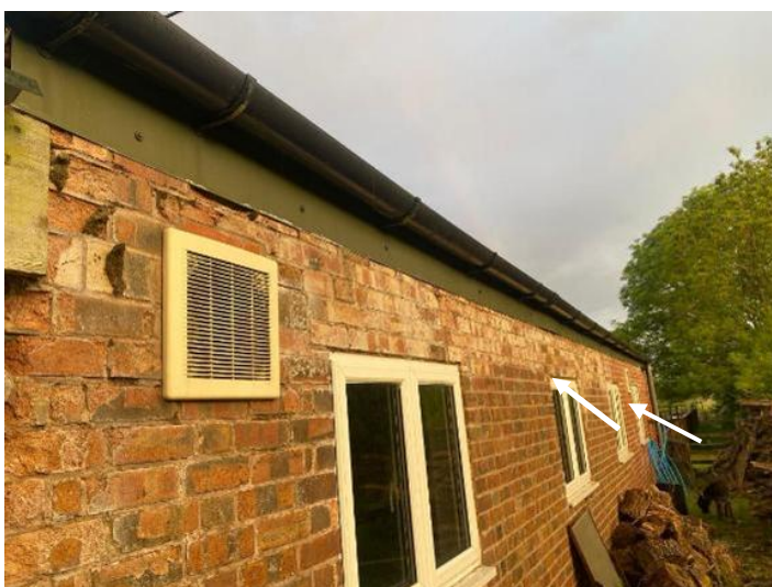
Photo 3. Facing northwest toward gaps above vent and under the bargeboard.
