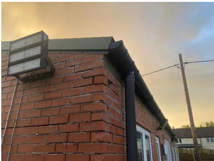
Photo 2. Loose half brick to the southeast corner with security lighting.
