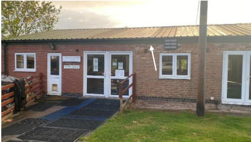
Photo 1. Facing northeast toward the hydrotherapy pool building showing the external lighting and area where the metal bargeboard is slightly lifted from the wall (arrowed).
