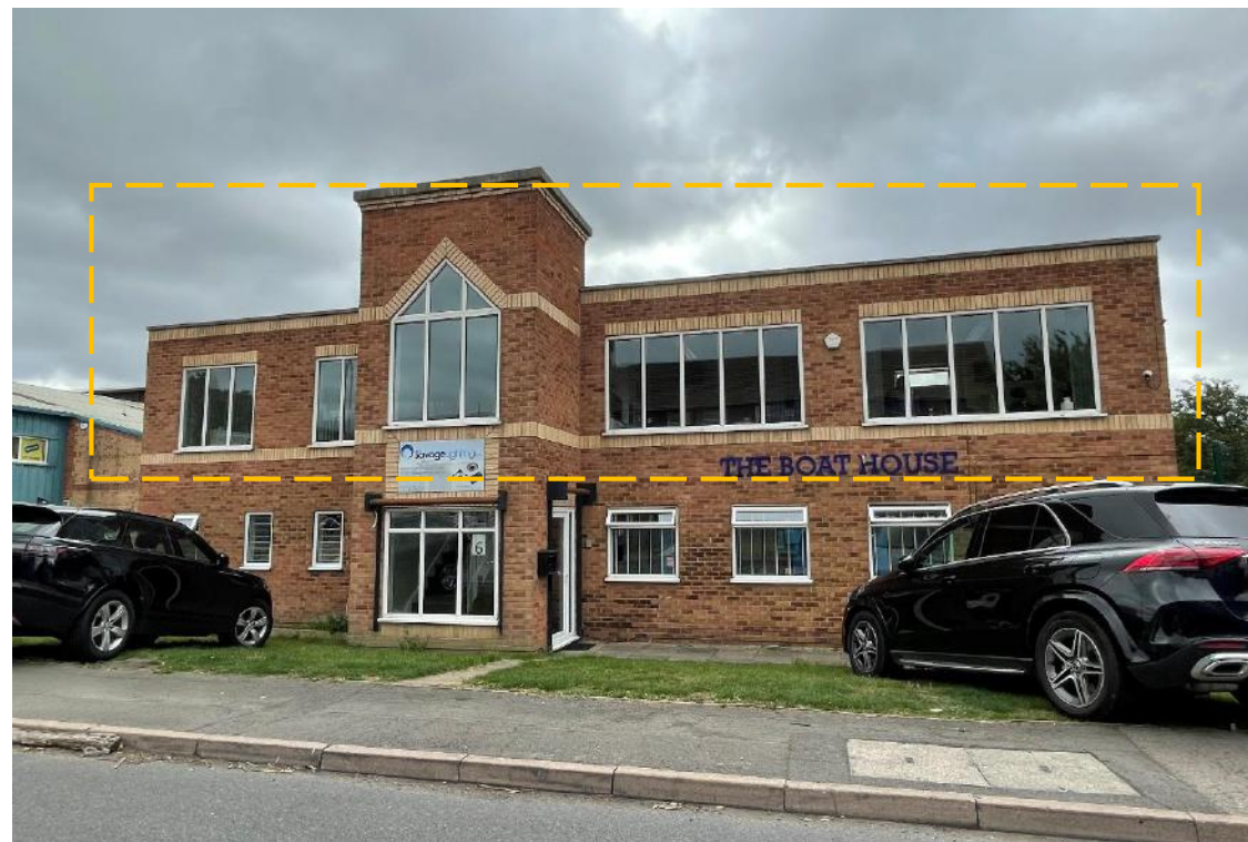
Offices (Savage Marine rent the first floor only)
