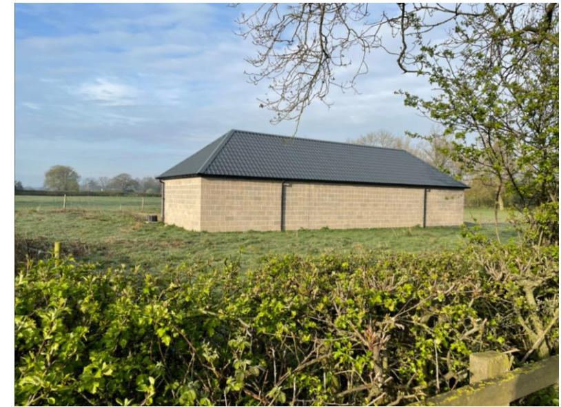
Adjacent stable building on Leicester Lane
