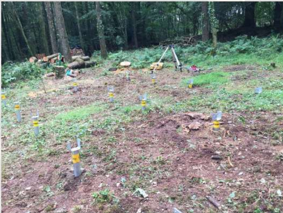
Screws installed ready for base frame
