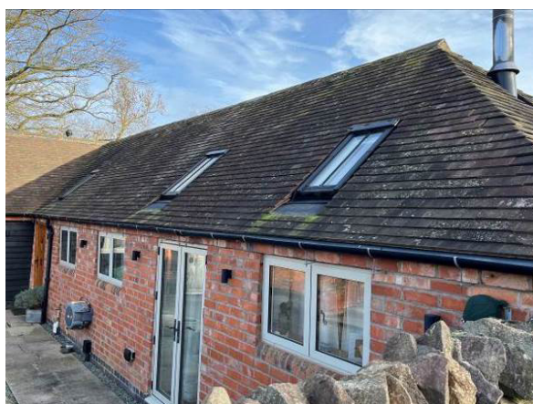
West facing roof structure
