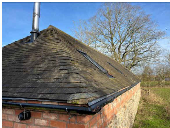
South and east facing roof structure
