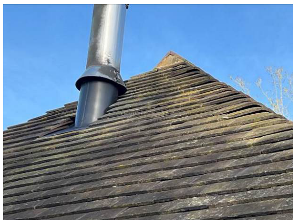
Close up of south gable roof and chimney
