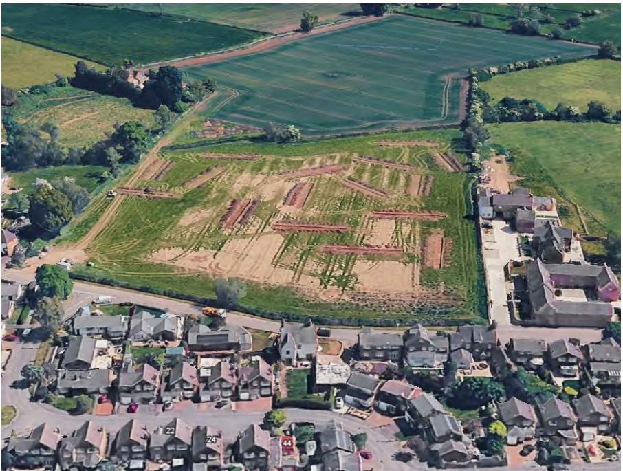
View from the West
