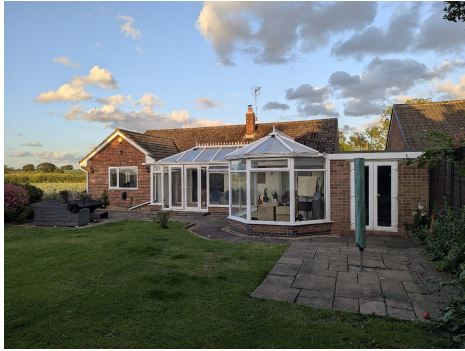
V1 B1-3 surveyor photo
