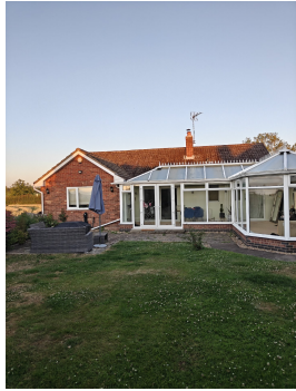
V2 B1-3 surveyor photo
