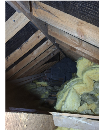
Figure 1a: Internal loft space North West
