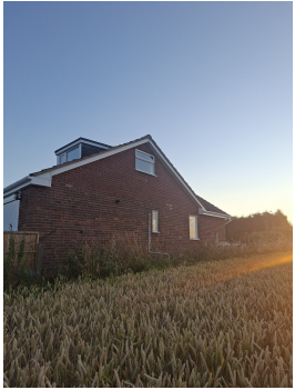
V2 B1-2 surveyor photo
