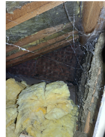
Figure 1b: Internal loft space South East
