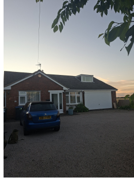
V2 B1-1 surveyor photo
