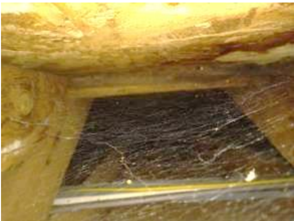
Plate A4.7: View into void in pitched roof space.
