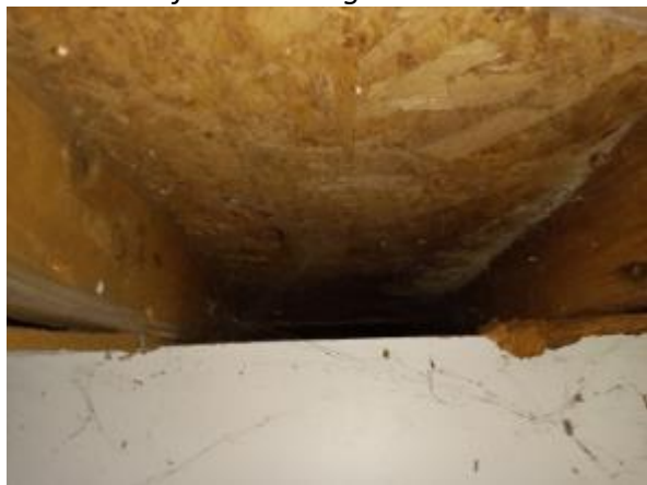
Plate A4.6: View into shallow void in sloping roof section.
