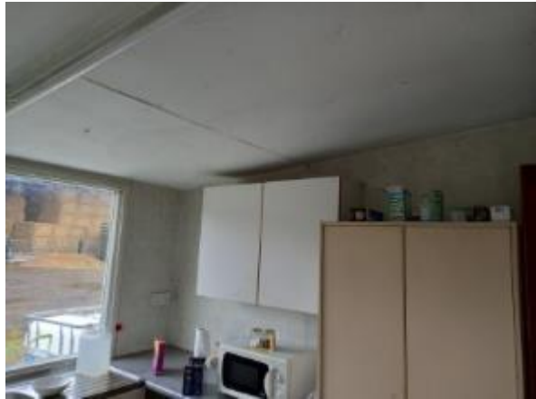
Plate A4.4: Sloping roof within kitchen on north side of the building.
