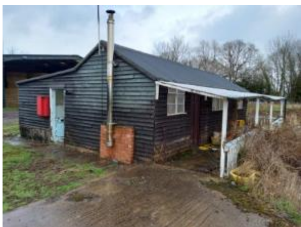
Plate A4.1: Bungalow – south and west elevations.
