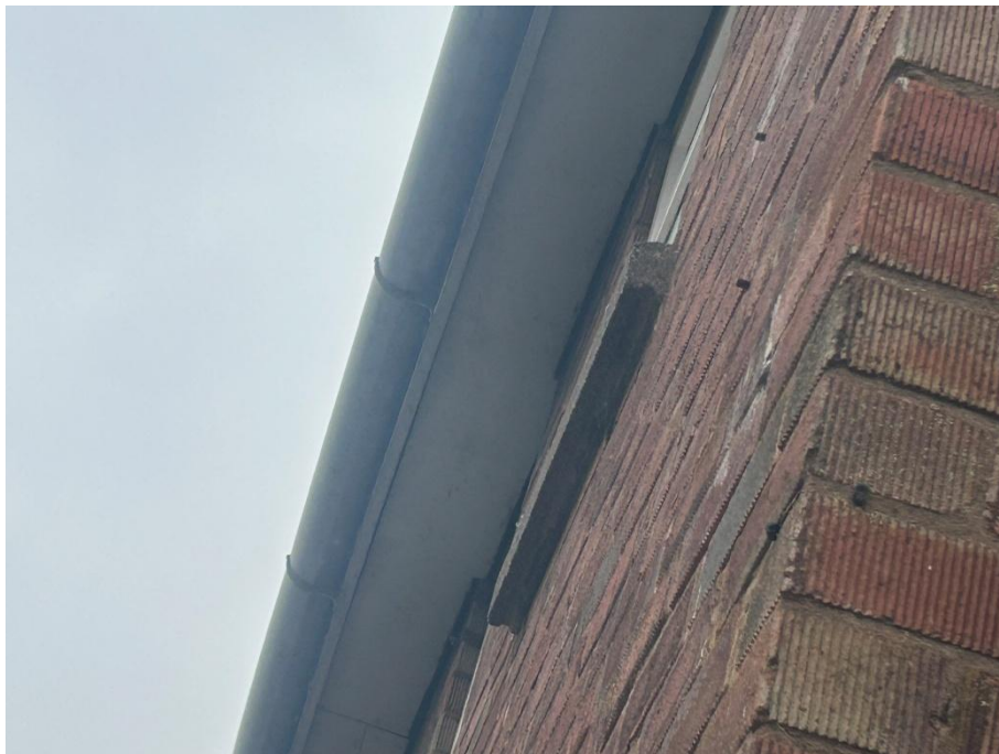
Photograph 5 – Narrow gap where the soffit meets the wall, but a very tight gap and no evidence of bats entering
