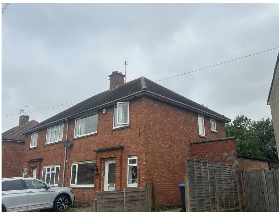
Photograph 2 – The south and east aspect of the property.
