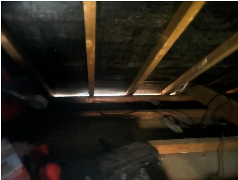
Photograph 9 – Light ingress from where the soffits meet the walls into the roof void but very tight gap and no evidence of bats entering
