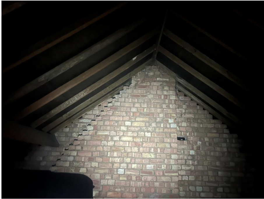
Photograph 8 – The internal loft space
