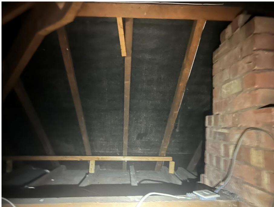
Photograph 11 – The internal loft space
