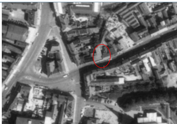
17 June 1959 Aerial View
