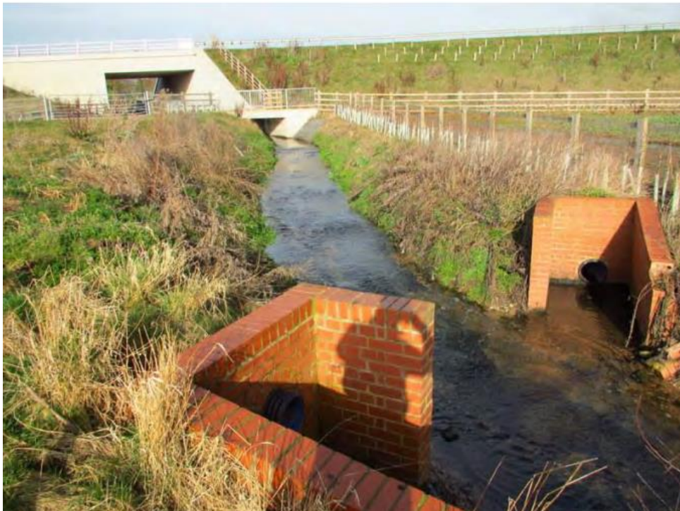
Plate 8– Earl Shilton Brook view upstream from east of A47 (structure 1 and A47 underpass at back of pictures). Outlet structures are associated with A47 bypass SuDS
